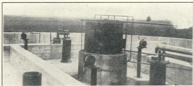
Floating Roof, Gas Dome, and Sludge Samplers on Digester
