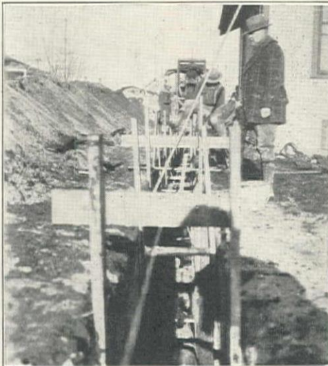
J. F. Shea & Co. Laying 15-in. Vitrified Pipe Intercepting Sewer at Klamath Falls. Gladding, McBean & Co. Pipe. Austin Trencher in Background
