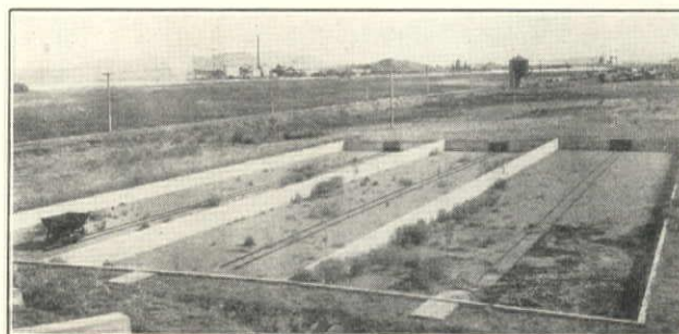
Sludge Drying Beds at Klamath Falls Plant
