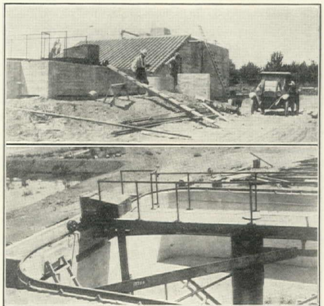
(Upper) General View of Sebastopol Sewage Treatment Plant. (Lower) Dorr Clarifier Equipment at Sebastopol
