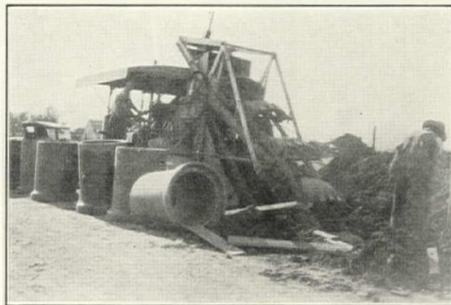
Gustine 24-in. Vitrified Pipe Outfall Sewer, John Pestana, Contractor
