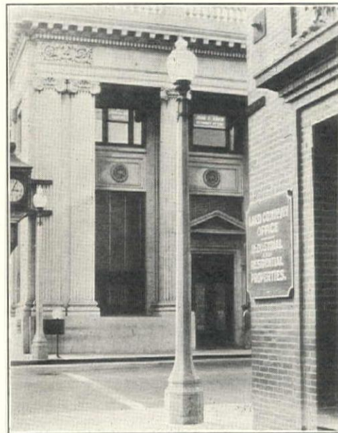
Recent Installation of Hollowspun Granite Lighting Standards in South San Francisco
