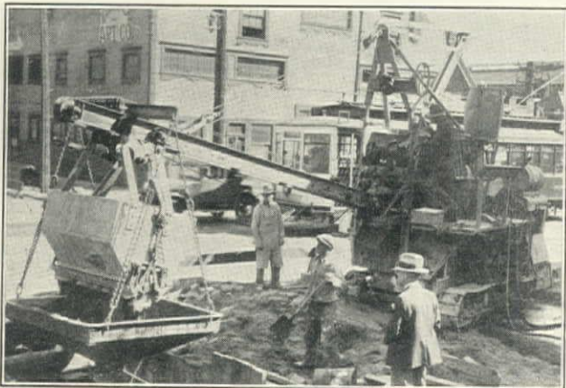
L. J. Cohn Placing Concrete on Section B, Fillmore St. Sewer, San Francisco, with MultiFoote Paver
