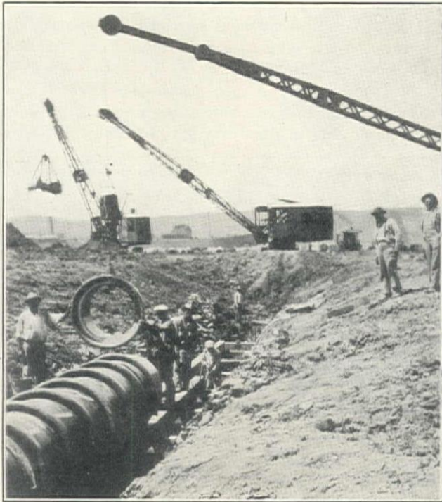
M. J. Bevanda Contract for Solano County Sewers, Showing 36-in. Vitrified Pipe Outfall and Two 1\frac{1}{4} -yd. Northwests and One \frac{3}{4} -yd. Buckeye. Line Rests on Piles, Bents Spaced 9 ft., Stringers 8 by 12 in.
