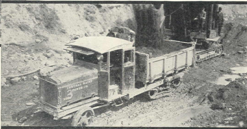
One of a fleet of fourteen Linn Tractors purchased by the Central Maine Power Co. of Augusta, Maine. They are being used in moving the 2,500,000 cubic yards of dirt involved in constructing the Wyman Dam at Bingham, Maine.
