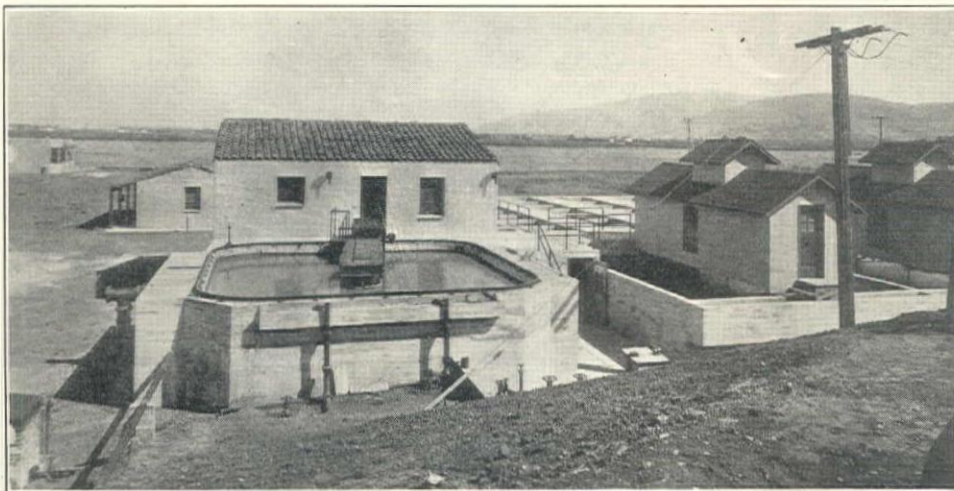
SALINAS SEWAGE TREATMENT PLANT, SHOWING PRIMARY CLARIFIER, BLOWER HOUSE, FINAL CLARIFIERS, AND AERATION BASINS
