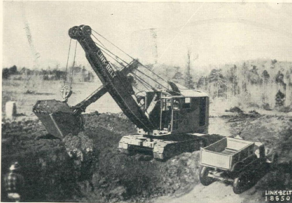
An average of 1,000 yards per 10-hour day is handled with one shovel and four 1-ton trucks.
