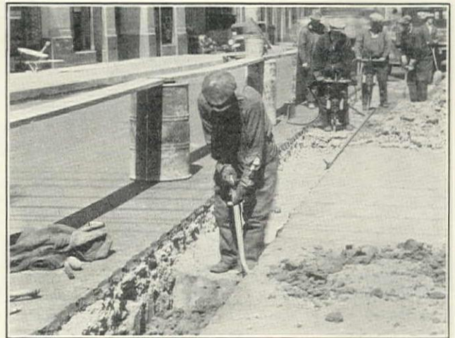
Two Rodax Pavement-Breaking Machines in Action
