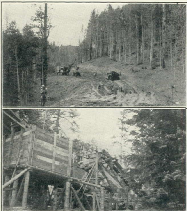
(Upper) Hodgman & McVicar Using Northwest 1-yd. Gas Shovel and 5-ton Autocar Trucks for Rough Grading Grand Canyon Route 4. (Lower) Lord & Bishop Crushing Plant for Surfacing Grand Canyon Route 3
