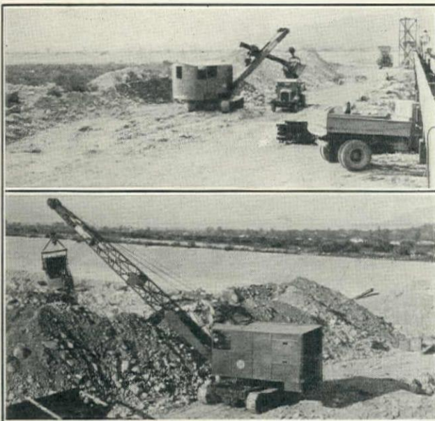
(Upper) Link-Belt ¾-yd. Gas Shovel Loading Backfill for Redwood Bents. (Lower) Link-Belt ¾-yd. Dragline Excavating Pier Footings
