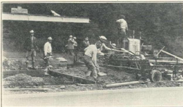
Pacific Highway Between Fort Lewis and Nisqually, Washington; Joseph L. Warter, Sr., Contractor. Laying Cement Concrete Pavement with MultiFoote Paver and Lakewood Finisher
