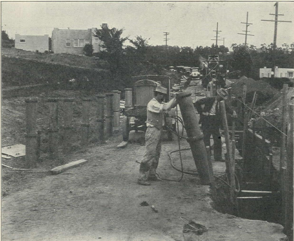
EDITH Street Sewer, Oakland. R. B. McNair, Contractor. For this installation of Vitrified Salt-Glazed Clay Pipe there was required 13,800 Ft. of 8" pipe and 406 Tees, Ys, etc. Sewers laid with such pipe will last indefinitely.
