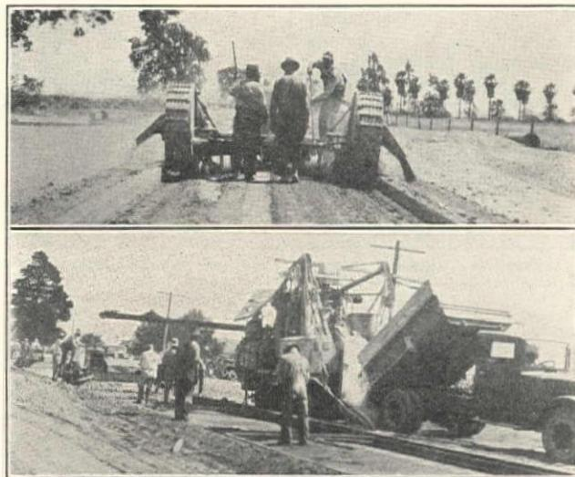
Reconstructing State Highway with Cement Concrete Pavement Between Cherokee Station and Harney Lane, San Joaquin County, California; T. M. Morgan Paving Co., Contractors. (Upper) Carr Subgrader with Clausen Tailing Elevating Wheels. (Lower) Koehring Paver Followed by Two Ord Finishers
