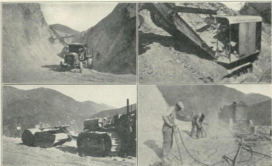
LA CANADA-MT. WILSON JOB—(UPPER LEFT) NORTHWEST 1½-YD. GAS SHOVEL CUTTING THROUGH HILL AT STA. 139+00; STERLING 7-YD. DUMP TRUCK IN FOREGROUND (UPPER RIGHT) THE W. LORAIN 1¼-YD. SHOVEL CAUGHT IN 4000-YD. SLIDE AT STA. 160+00; SHOVEL SHOVED TO EDGE OF 200-FT. CLIFF AND OPERATOR REMAINED AT THE LEVERS WITHOUT INJURY (LOWER LEFT) CATERPILLAR '60' AND McMILLAN SCRAPER (LOWER RIGHT) INGERSOLL-RAND EQUIPMENT FOR DRILLING
