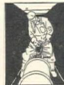
And in addition it has unusual adhesion and is flexible enough to allow normal or even extreme movement of lines in settling without damage to joints. Ric-wil Compound is economical and easy to pour.
