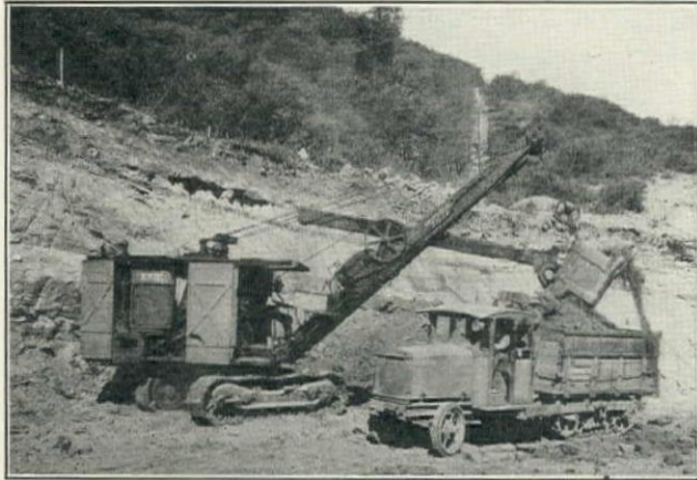
Bucyrus-Erie 1 1/4-yd. Gas+Air Shovel Loading 8-yd. Republic-Linn Truck Tractor on Sepulveda Blvd.
