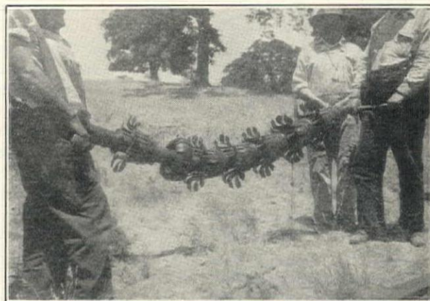
Fig. 2. Pontoon (or Mushroom) Type Cleaner Used by National Water Main Cleaning Co. on Recent Stanford University Contract
