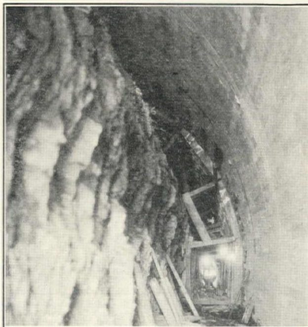
Side Drift and Concrete Lining for Sepulveda Tunnel, Wall Forms Braced from Central Core
