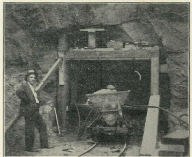
Starting East Drift from North Portal, Sepulveda Tunnel, J. G. Donovan Standing Near 16-ft. Koppel Type Muck Car. Two Douglas Fir Sets in Place
