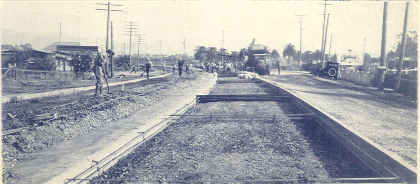
PLACING ASPHALTIC CONCRETE AND PORTLAND CEMENT CONCRETE ON 8.7-MILE SECTION OF CALIFORNIA STATE HIGHWAY BETWEEN HAYWARD AND NILES, HANRAHAN CO., CONTRACTOR
