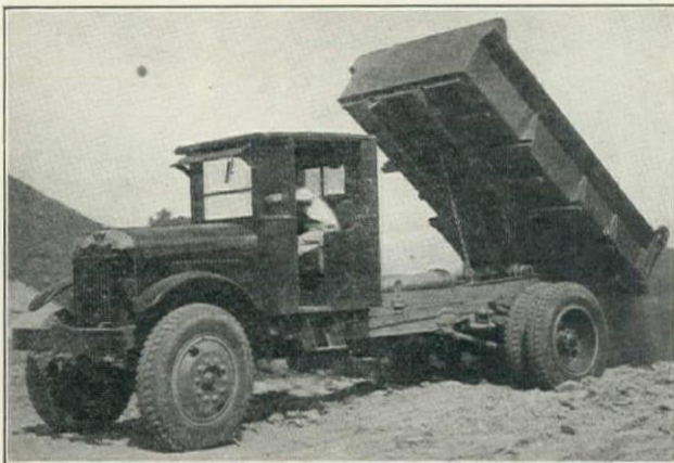
Republic 4-yd. Dump Truck Grading on Sepulveda Blvd.
