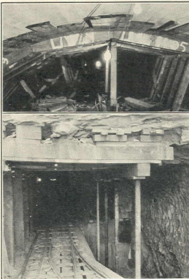
(Upper) Timbering and Forms in Top Drift Near South Portal. (Lower) Pipe Sprags Carrying Load on Side Drift
