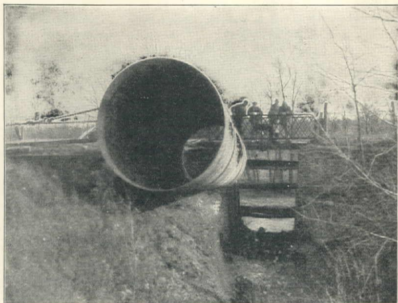
A 96-inch Armco Culvert Bridge replacing a structure that had become obsolete and unsafe.
