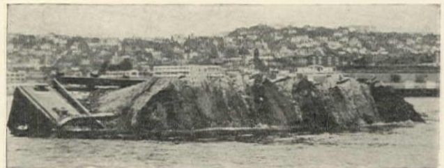
Reversible Scow Discharging 400-cu.yd. Load in Elliott Bay
