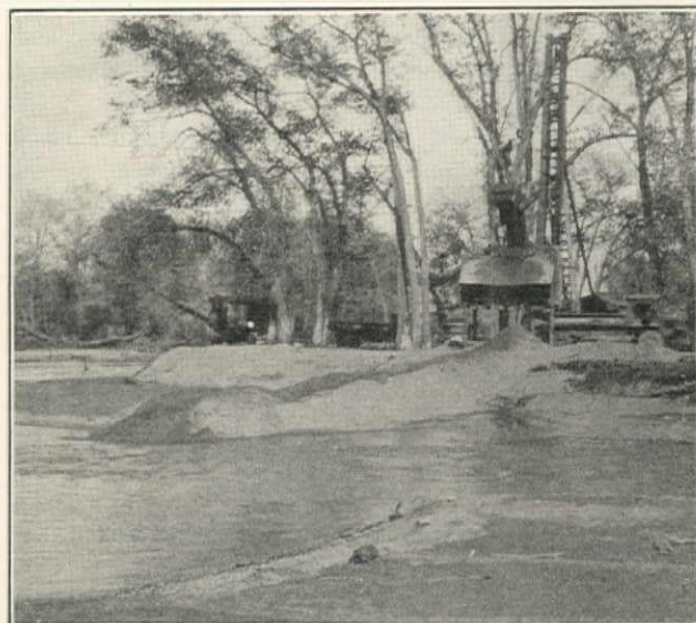
Speeder \frac{1}{2} -yd. Dragline and Sauerman 1-yd. Cableway Bucket Taking Pit-Run Material from Platte River, Englewood-Littleton Highway
