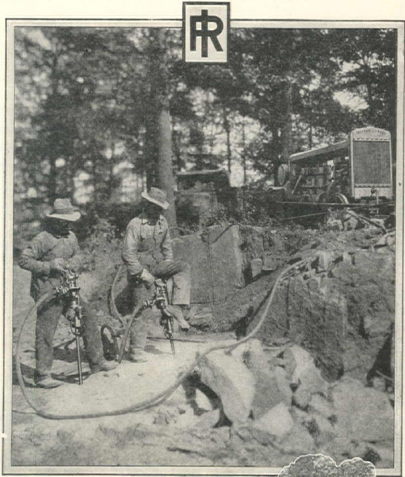
Above: "Jackhamer" Drills at work on a road-building project. Below: Truck-mounted Portables furnishing air to "Jackhamer" Drills in excavation work.
