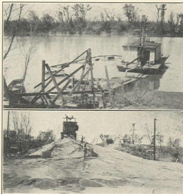
American River Bridge for Sacramento County, California, Lord & Bishop Contract, Showing Intake and Discharge for Sand Fill on Approach
