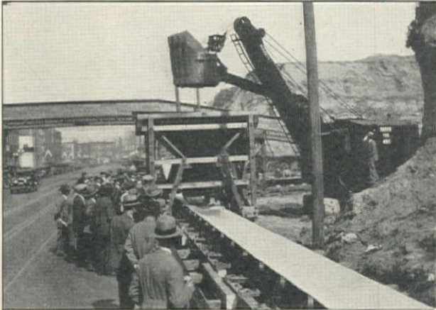
Marion 2-yd. Electric Shovel Near Central Collecting Point for Denny Hill Regrade No. 2
