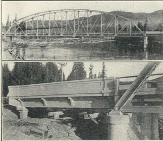
Priest River Bridge for Idaho Bureau of Highways, May 11, Showing Main Steel Span and Details of Concrete Approach Span, Sam Boudrye Contract
