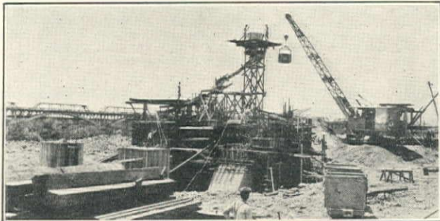
Salt River Bridge at Tempe for Arizona Highway Department, Lynch-Cannon Engineering Co. Contract. Link-Belt Type K-2 Crane and 30-cu.ft. Containers Placing Concrete in 4-cu.yd. Batches for Cap of South Abutment
