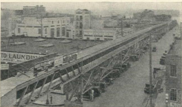
Overhead Conveyor on Battery St., Showing Substantial Housing, Denny Hill Regrade No. 2
