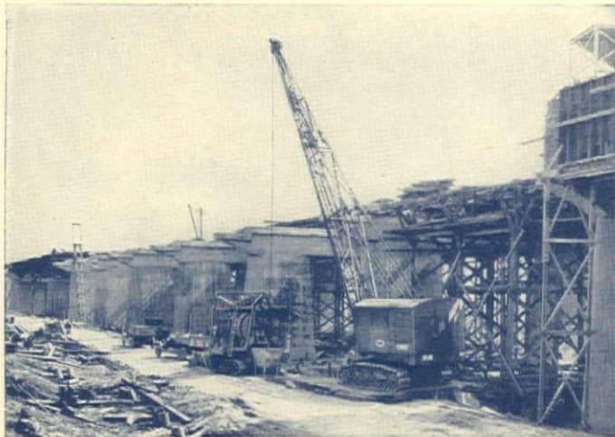
P & H Model 600 Corduroy Crane placing concrete on Commerce Street viaduct job, Dallas, Texas.
