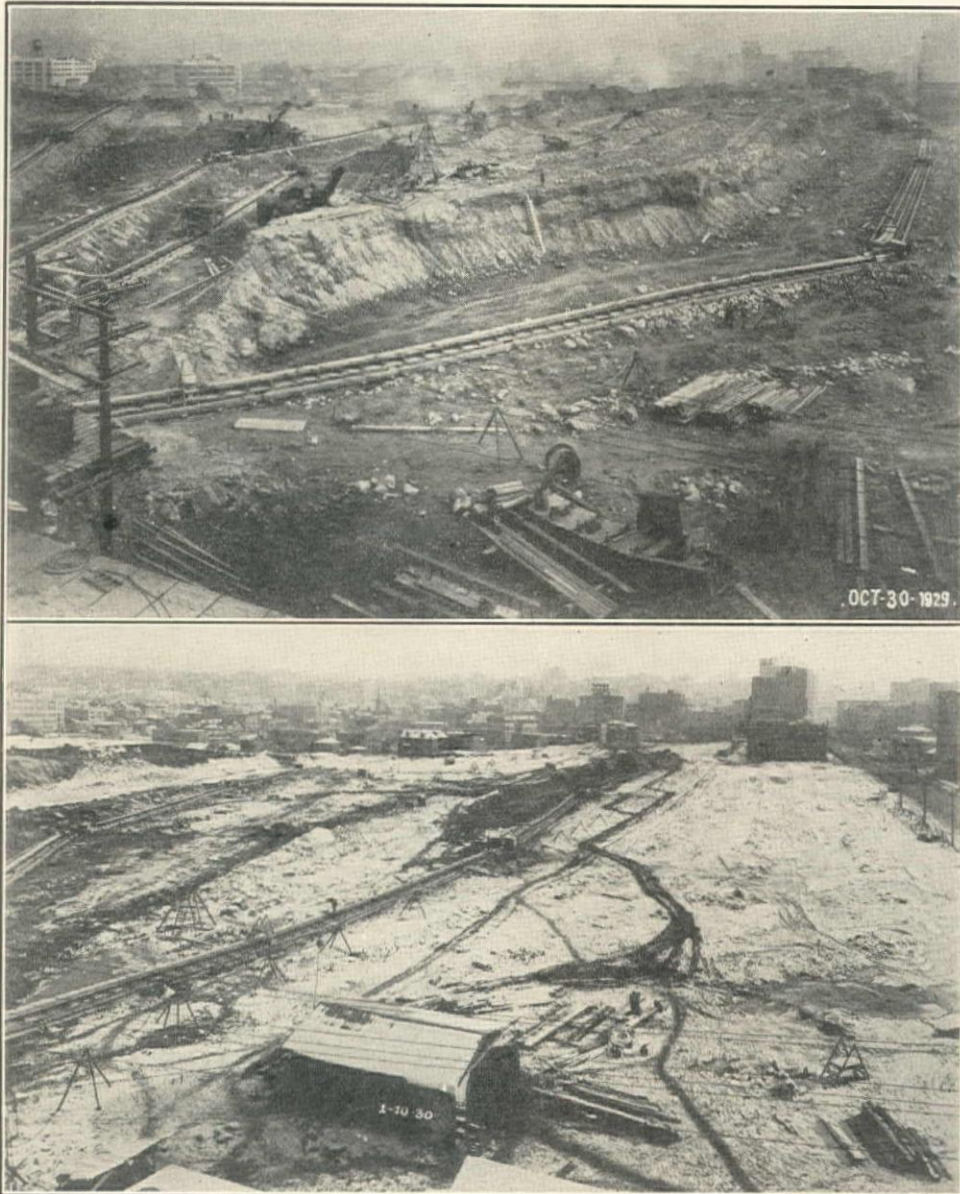
BATTERY OF 2-YD. MARION ELECTRIC SHOVELS DISCHARGING INTO PORTABLE STEEL HOPPERS AND THENCE TO MOVABLE BELT SECTIONS. DENNY HILL REGRADE No. 2 ON OCTOBER 30, 1929, AND JANUARY 10, 1930
