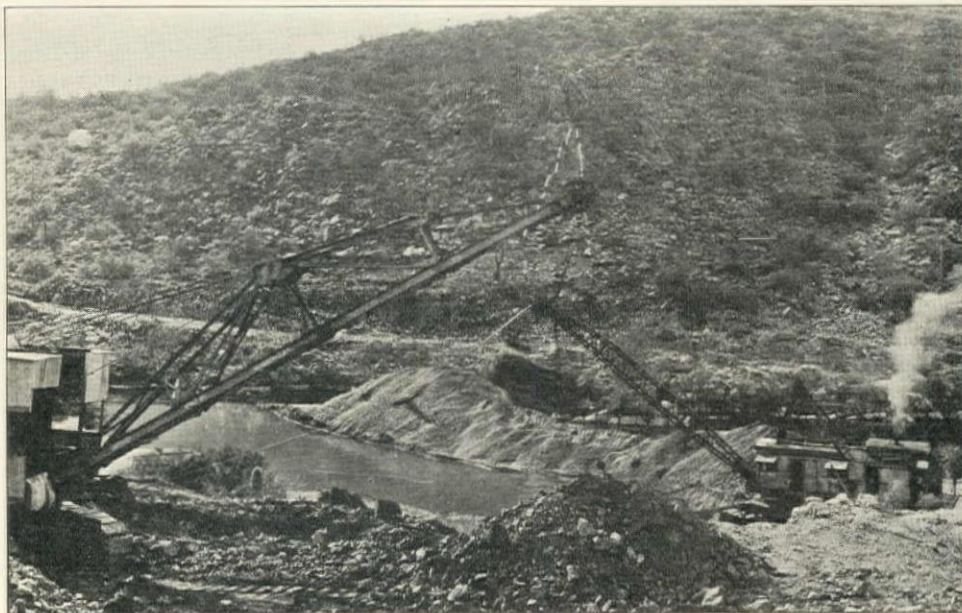
BUCYRUS \frac{2}{2} -YD. DRAGLINE AND P&H \frac{1}{2} -YD. DRAGLINE EXCAVATING FOUNDATION FOR STEWART MOUNTAIN DAM
