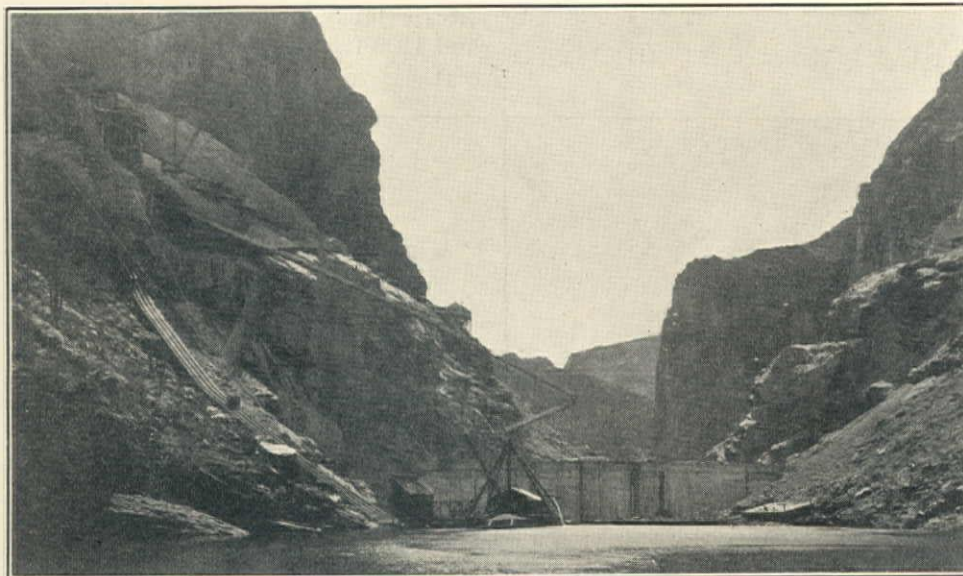
HORSE MESA DAM, SEPTEMBER 14, 1926, FROM UPSTREAM. GRAVEL SCOW BEING UNLOADED. INCLINED TRACK, CONCRETE MIXING PLANT, AND PLACING EQUIPMENT IN LEFT FOREGROUND
