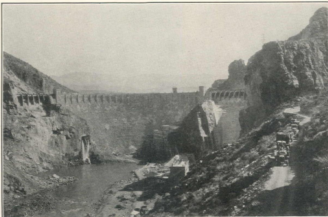
ROOSEVELT DAM AND POWERHOUSE FOR THE SALT RIVER VALLEY WATER USERS' ASSOCIATION, COMPLETED (BY U. S. GOVERNMENT) IN 1911 WITH SUPPLEMENTAL WORK IN 1913 AND 1923, HEIGHT 284 FT., GENERATING CAPACITY 24,000 HP., STORAGE 1,637,000 AC-FT. THREE NEEDLE VALVES HAVE BEEN REMOVED
