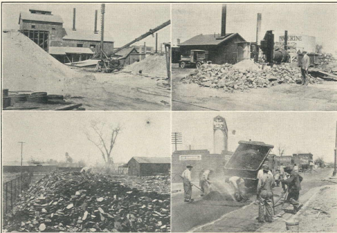
(UPPER LEFT) MAIN ASPHALT PLANT OF DENVER DEPARTMENT OF IMPROVEMENTS AND PARKS. (UPPER RIGHT) EQUIPMENT FOR RECLAIMING USED ASPHALT FROM DENVER STREETS. (LOWER LEFT) SORTING OLD ASPHALT ON STORAGE PILE. (LOWER RIGHT) MAKING A LARGE PATCH ON A DENVER STREET
