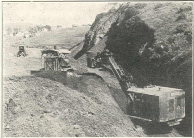
Marion 1 1/4-yd. Electric Shovel and Caterpillar with Bulldozer on Section 'A' of Aleman Storm Drain, S.bley Grading & Teaming Co. Subcontract
