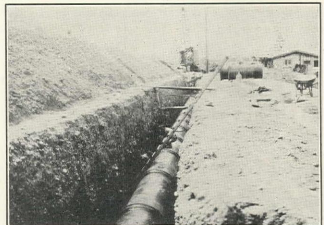
Miracle Construction Co. Laying 36-in. Cast-Iron Pipe (U. S. Pipe & Foundry Co.) on Schedule 4, Otay Reservoir-San Diego Second Main Pipe-Line
