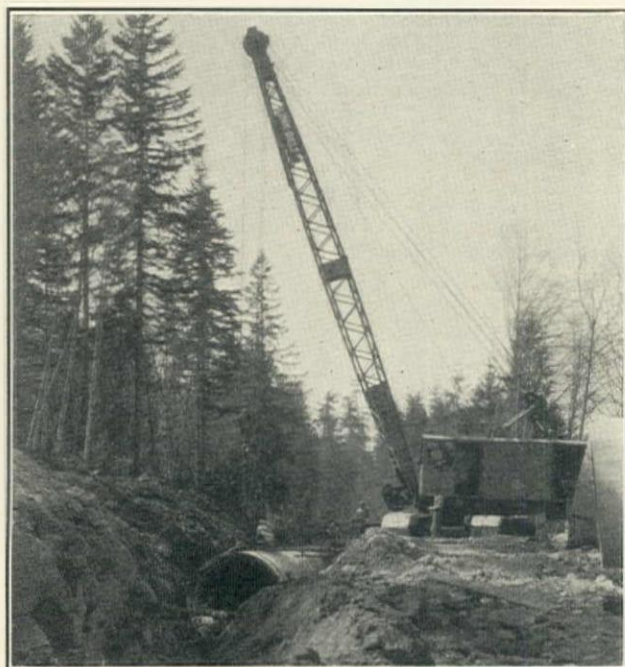
Link-Belt K-55 Crane Laying Section of 96-in. Precast Concrete Pipe Weighing 42,000 lb. for Lake Youngs Aqueduct, Seattle, Elliott, Stroud Bros. & Seabrook Contract
