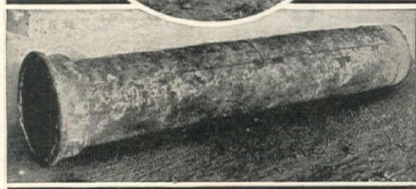
Top: 10" cast iron pipe laid at Portage, Wis., in 1887, taken up in perfect condition and relaid. Below: Cast iron pipe laid at Philadelphia, Pa., in 1819, removed during South Broad Street Subway excavation and found in perfect condition.
