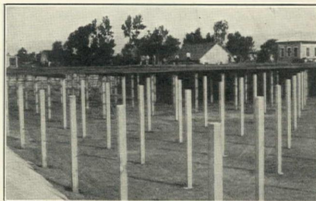
Placing Redwood Roof on Cast-in-Place Concrete Piers for Reservoir No. 1 Near Freedom Village, Watsonville Water Improvements
