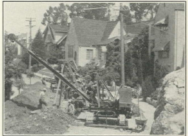
Austin Model BF-4 Backfiller Following Austin Model 42-15 Trencher on J. C. Hickey Contract for Unit 4 of Berkeley Storm Drain System
