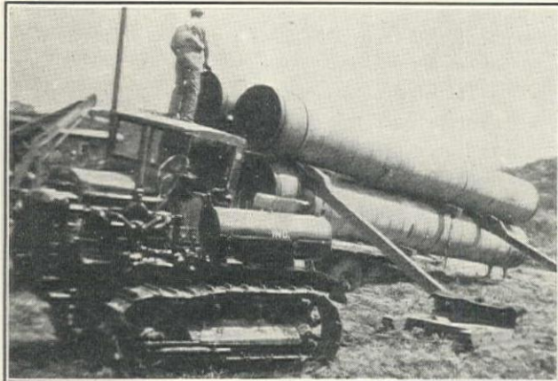
Western Pipe & Steel Co. Unloading 36-in. Electric-Welded Steel Pipe on Schedule 2, Otay Reservoir-San Diego Second Main Pipe-Line
