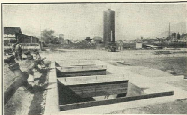
Clarifier, Suction Piping, and Scum Drain for Sebastopol Sewage Treatment Plant, A. F. Anderson, Contractor
