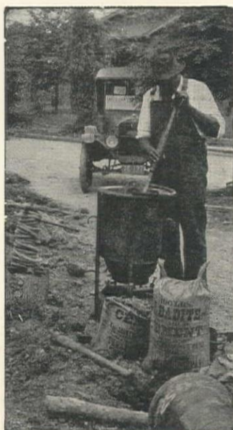
Melting Leadite prior to pouring joint.
