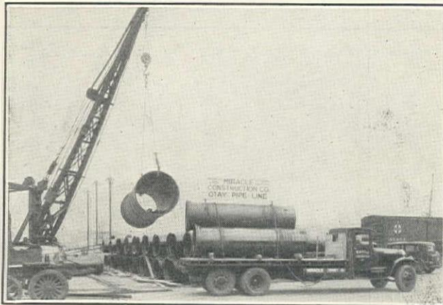
Pipe Yard of Miracle Construction Co., Contractor on Schedule 4, Otay Reservoir-San Diego Second Main Pipe-Line. Crane Handling Section of 36-in. Cast-iron Pipe Furnished by U. S. Pipe & Foundry Co.
