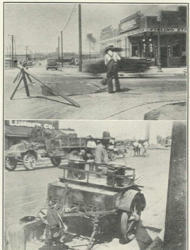
(Upper) Trenching and Filling Sunken Surface with New Topping. (Lower) Patching Crew at Work Cutting Out Damaged Pavement. Oil-Burning Tool Heater in Foreground
