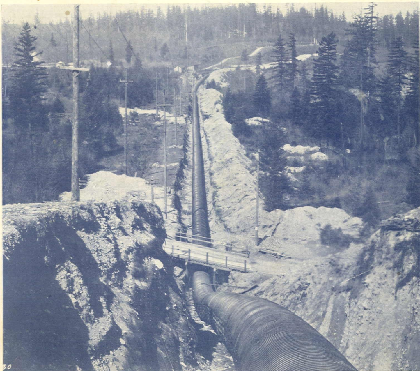
30 CEDAR RIVER PIPE-LINE No. 4 FOR SEATTLE WATER SUPPLY, SHOWING SECTION OF HANS PEDERSON CONTRACT FOR 54,500 LIN. FT. OF 78-IN. CREOSOTED WOOD-STAVE PIPE, BETWEEN WEST PORTAL OF LAKE YOUNGS AQUEDUCT AND EXISTING LINES NEAR MOLASSES CREEK CONTROL WORKS
