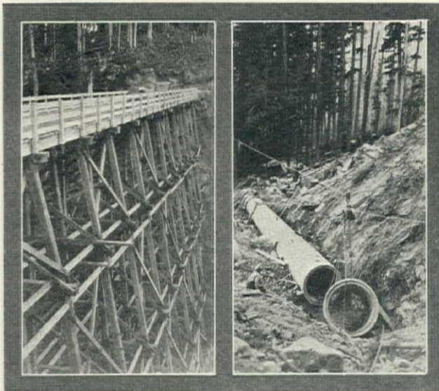
(Left) Timber Trestle Bridge 90 ft. High Over Deadwood Creek, Von der Hellen & Pierson Contract. (Right) Placing 60-in. Extra Strength Reinforced Concrete Pipe by Means of Chain Blocks and Highline, Von der Hellen & Pierson Contract, Morse Creek to Crystal Creek
