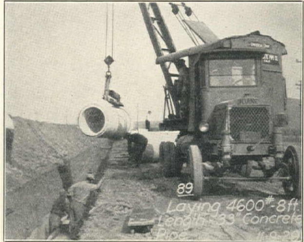
Universal Crane Laying 33-in. Hume Concrete Pipe for Supply Main from Mallard Pump Station to Chenery Reservoir, November 9, 1929
