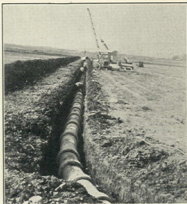
Hume 33-in. Concrete Pipe-Line from Mallard Pump Station to Chenery Reservoir, Universal Crane in Distance
