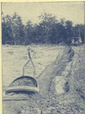
Digging Material for Levee
