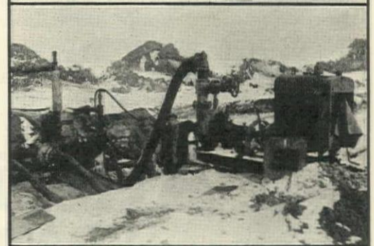
Illustration shows three F-M Wood Trash Pumps in operation.
