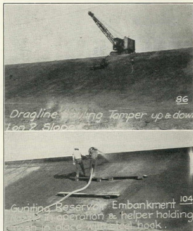
Completing Inside Slope of Chenery Reservoir Embankment
