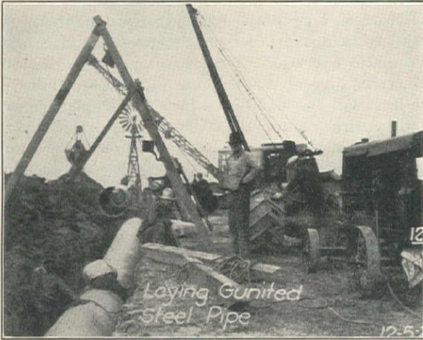
Laying 36-in. Electric Welded, Gunite Coated, Steel Pipe, near Mallard Pump Station, December 5, 1929
