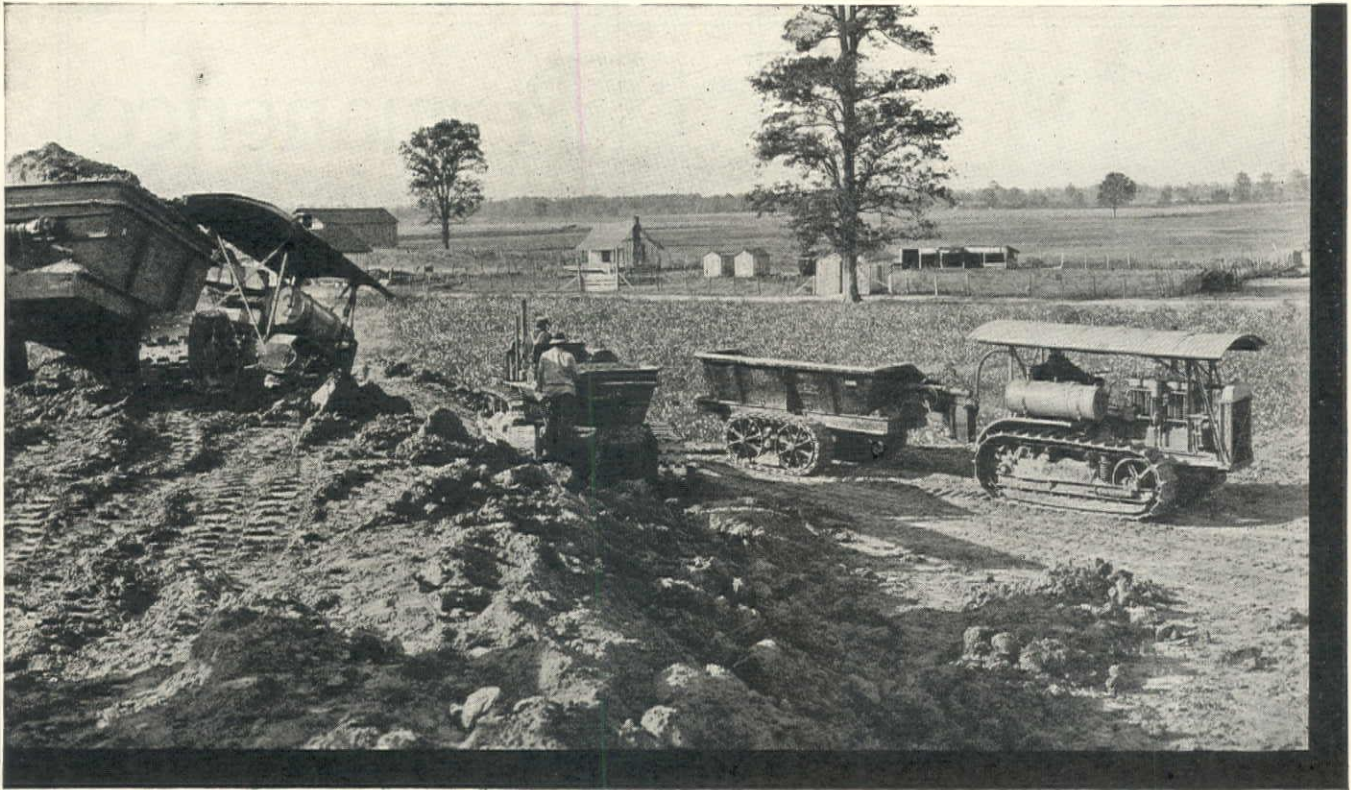
*Building a levee on the Mississippi River at Pecan Point, Arkansas (S. A. Hunter Co.)
