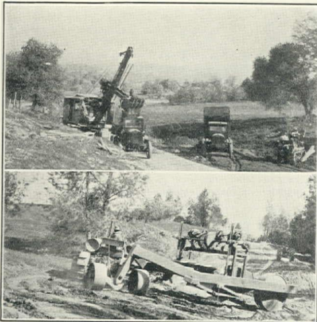
(Upper) Northwest 1-yd. Shovel Loading Kleiber 5-yd. Dump Truck on Detour Near Calaveritas Creek, Larsen Bros. Contract, California Division of Highways. (Lower) Caterpillar '60' and Le Tourneau Scarifier on Larsen Bros. Contract in Calaveras County
