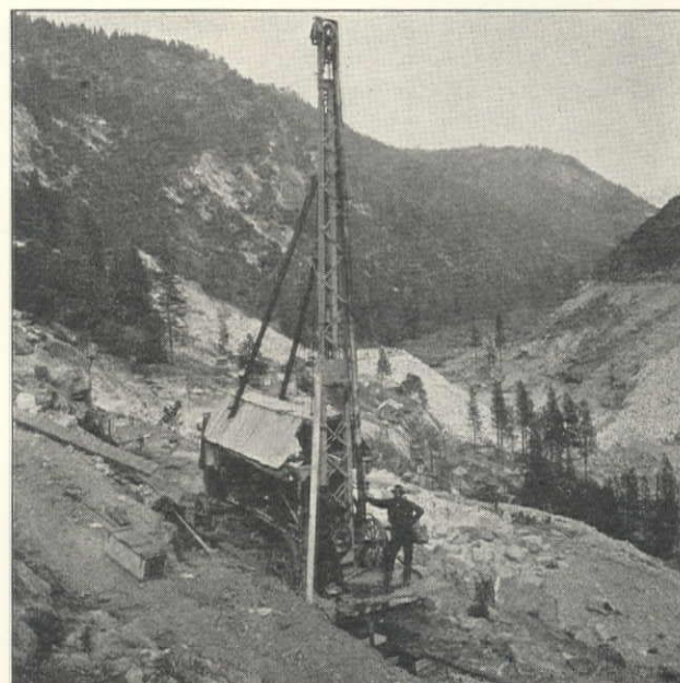
One of Five Armstrong Churn-Drill Rigs Drilling 5\frac{3}{4} -in. Holes 150 ft. Deep in Main Quarry for Salt Springs Dam
