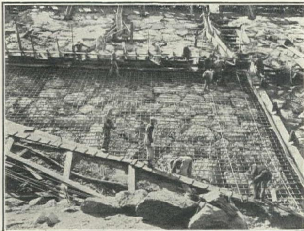
Salt Springs Dam. Placing Reinforcing Steel for Lowest Tier of Concrete Panels for Upstream Facing; Also, Pouring Footings Along Edges of 60-ft. Panels
