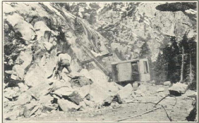
Northwest ¾-yd. Shovel and Drilling Equipment on Nate Lovelace Contract Near Bay View Rest, El Dorado County, California Division of Highways
