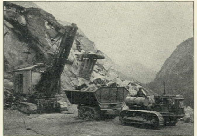
Salt Springs Dam. Marion 2-yd. Electric Shovel Loading Athey 20-ton End-Dump Trailer Truck Drawn and Powered by Caterpillar 60 Tractor, in Spillway-Cut Quarry
