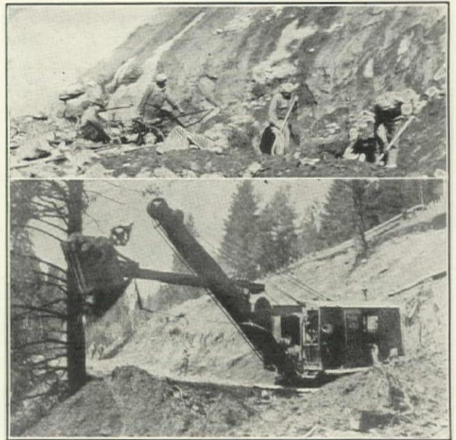
Tiger Creek Conduit, April, 1930. Drilling Base of Slope on 18-ft. Bench for Concrete and Side-Casting with Marion Type 450 Gas Shovel Near Tiger Creek
