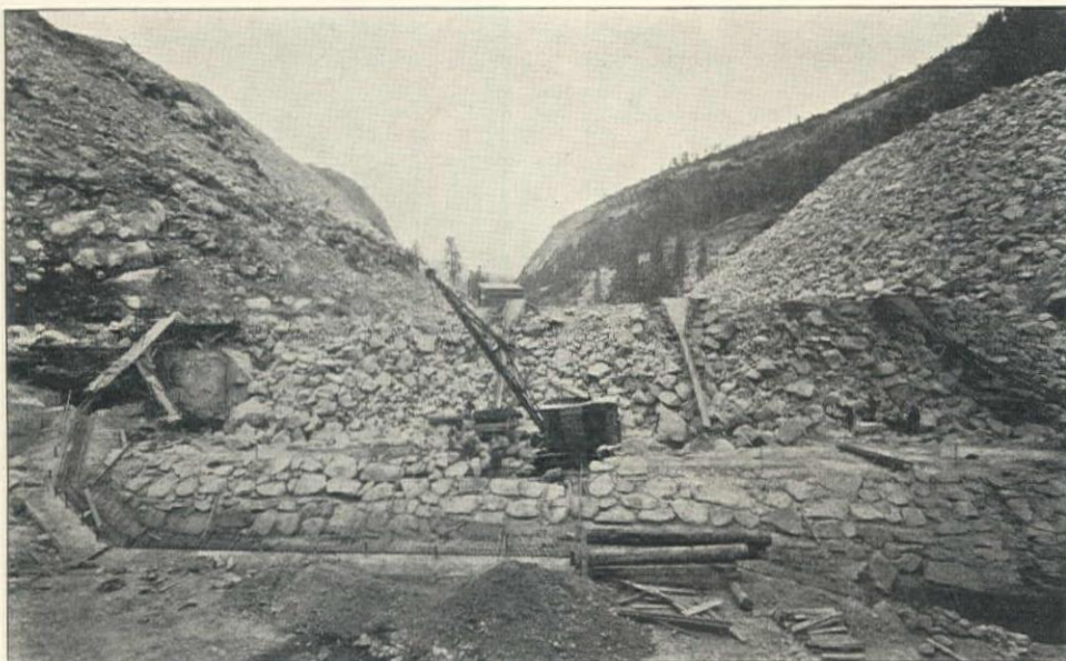
SALT SPRINGS DAM, LOOKING DOWNSTREAM, IN MARCH, 1928, SHOWING CUT-OFF WALL, BASE COURSE OF CRANE-PLACED ROCK SET IN CEMENT MORTAR, AND GROUT HOLE PIPES
