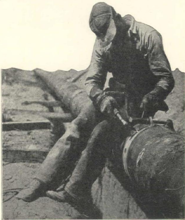
The welder is joining two sections of an Armco INGOT IRON pipe line installed for the cities of Woods Cross and Scipio, Utah. Pipe of four different diameters was used: 14-inch, 12-inch, 10-inch and 8-inch. Fabricated by the Burnham Manufacturing Company.
