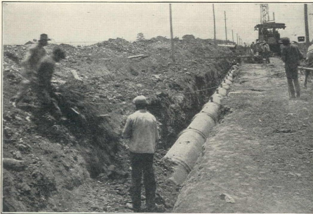
Laying 36 in. c.i. pipe with LEADITE Joints. Note that back-filling is immediately following the laying
