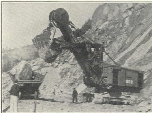
Salt Springs Dam. Bucyrus-Erie 120-B, 4-yd. Electric Shovel In Main Quarry Loading Railroad Car Equipped with End-Dump Body
