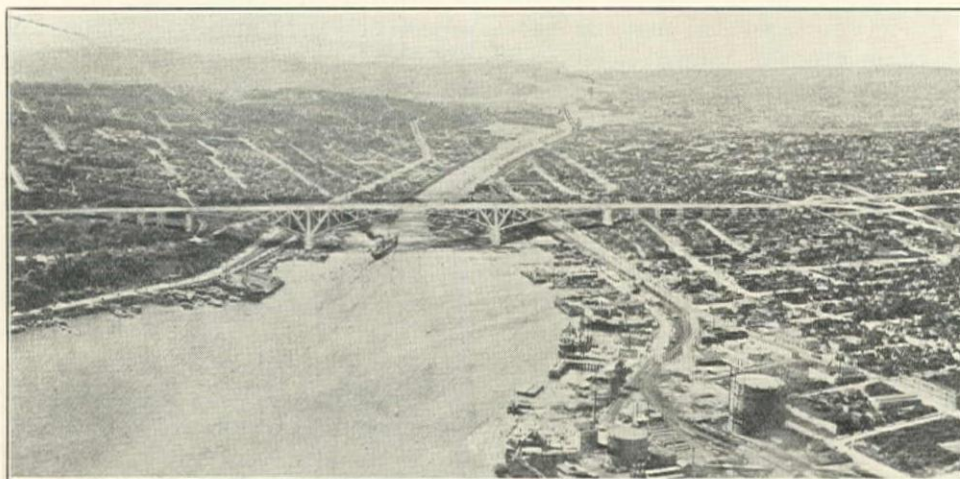
FIG. 1. CANTILEVER ARCH STUDY FOR AURORA AVE. CROSSING, LAKE UNION BRIDGE
