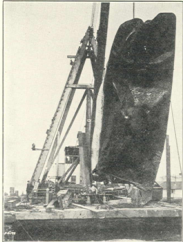
Derrick Scow 'Ajax' Holding Locomotive Tender Tank Pulled from Under Sheet Piling for Pier S1, Lake Union Bridge
