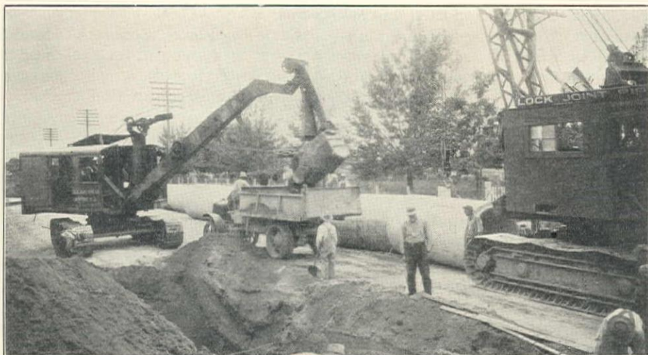
NORTHWEST 1\frac{1}{4} -YD. PULL SHOVEL AND WHITE TRUCK TRENCHING FOR CONDUIT NO. 13, CITY OF DENVER
