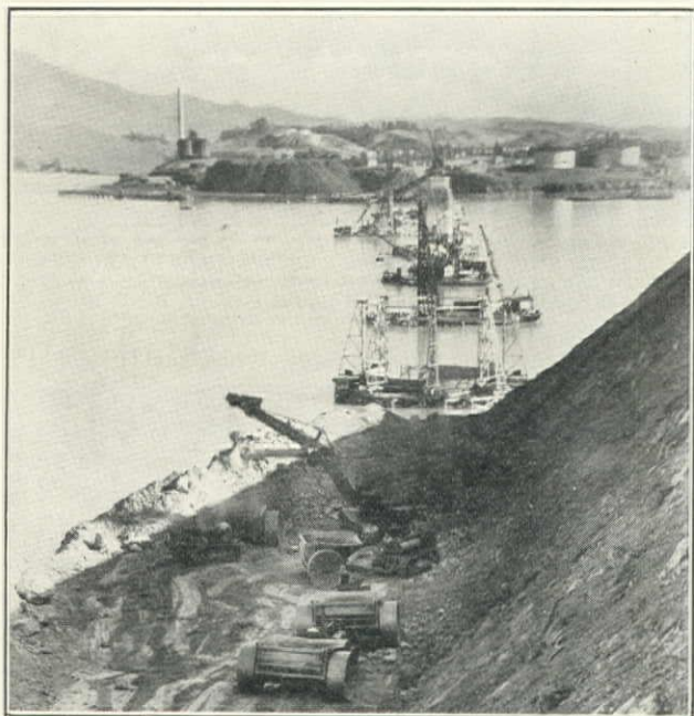
Bucyrus-Erie 50-B Diesel-Powered Shovel, Caterpillar '60's', and Le Tourneau 16-yd. Dump Wagons Completing 75-ft. Cut at Bridgehead. Main Piers (Siems, Helmers & Schaffner Contract) in Background
