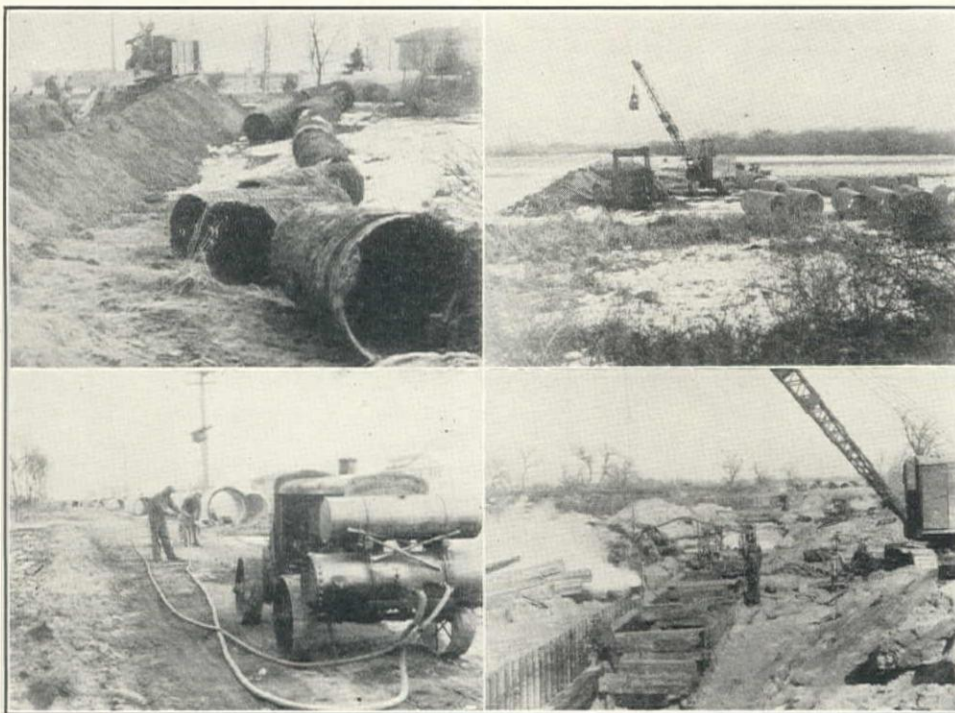
(UPPER LEFT) REMOVING OLD 48-IN. REDWOOD WOOD-STAVE PIPE. (UPPER RIGHT) PLACING 15-FT. SECTION OF TIMBER SHORING IN TRENCH THROUGH PLATTE RIVER BOTTOM. (LOWER LEFT) INGERSOLL-RAND 8 BY 6-IN. PORTABLE COMPRESSOR AND TWO DRILLS WORKING IN FROZEN GROUND. (LOWER RIGHT) DRIVING INTERLOCKING STEEL SHEET PILING FOR CHERRY CREEK CROSSING
