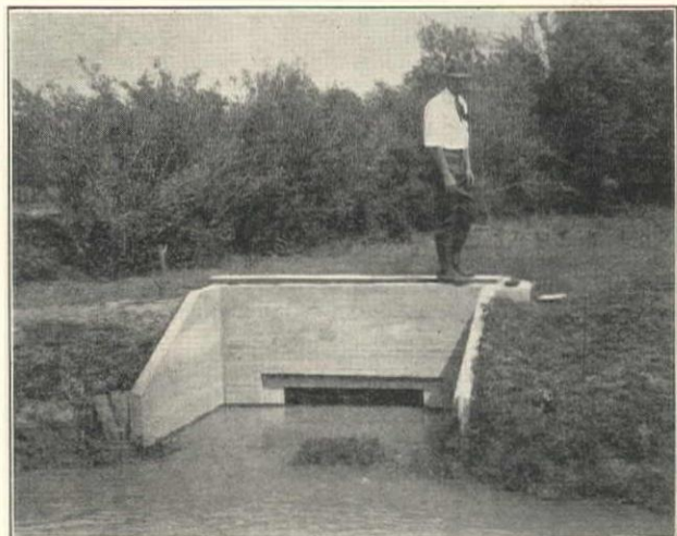
Great Western Meter Installation on 6 sq.ft. Orifice from Main Canal to Large Lateral
