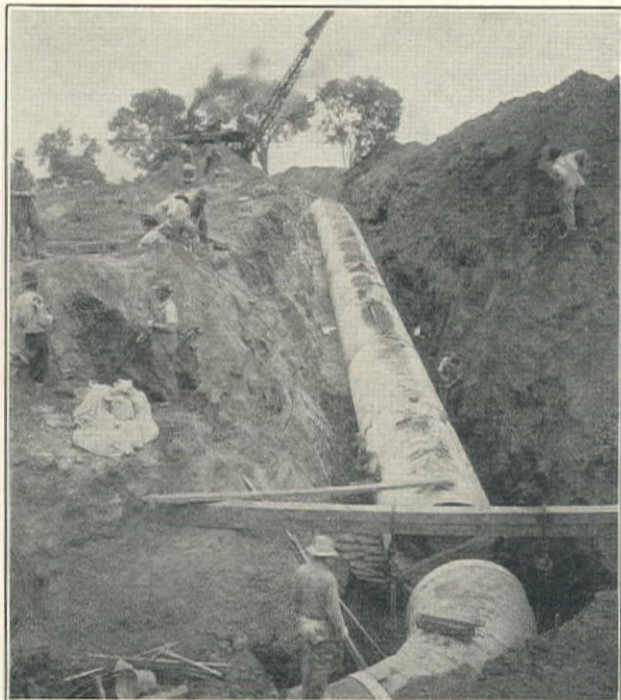
Pipe in Place for Closeup Section on Conduit No. 13
