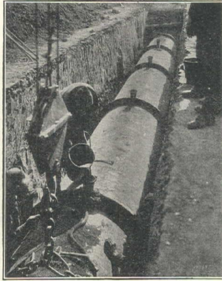
—Pouring 48-in. c. i. pipe joints with LEADITE
