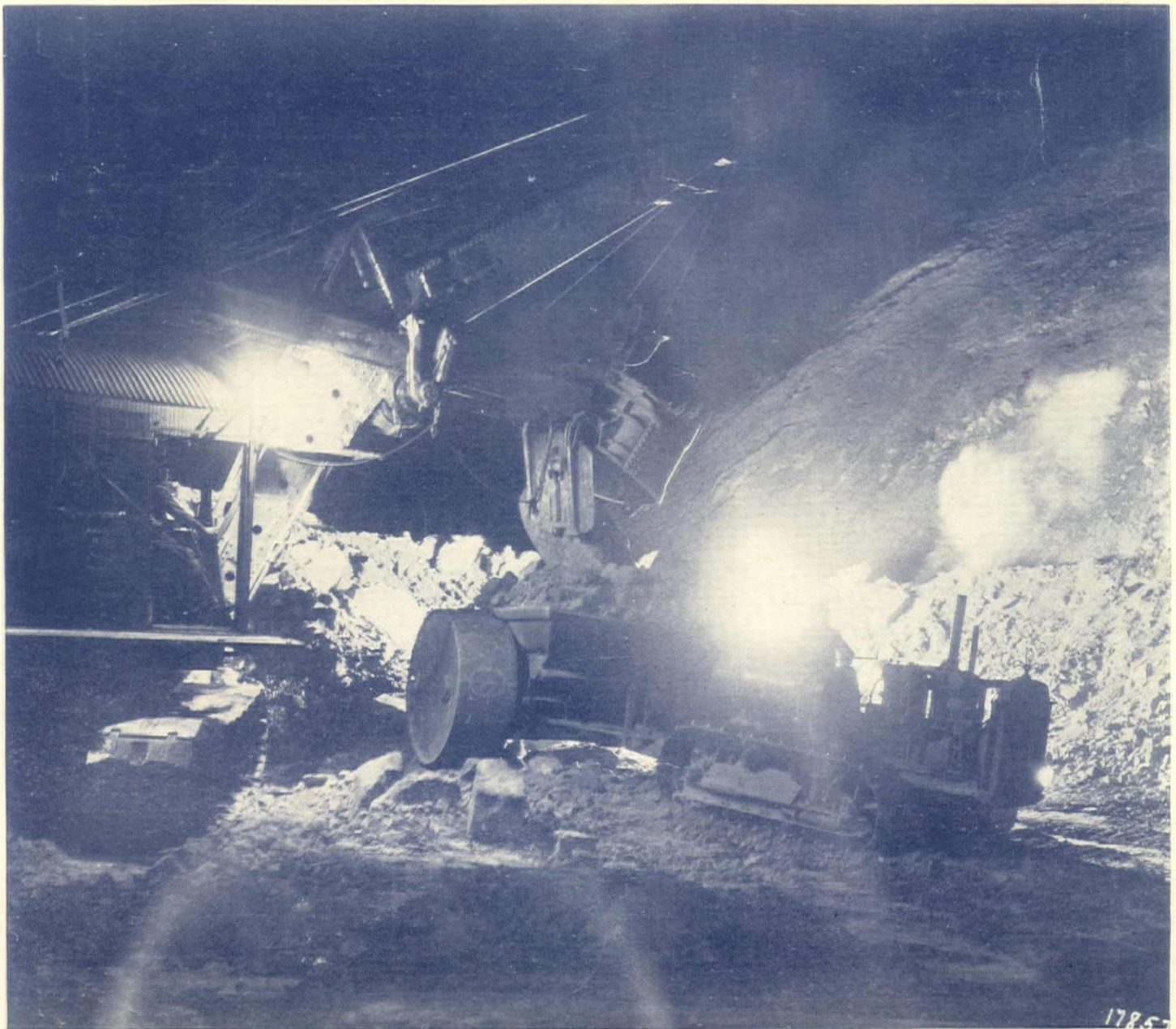
1785 DIESEL-POWERED 2-YD. SHOVEL, 16-YD. DUMP WAGON, AND 60-HP. TRACTOR IN HEAVY CUT ON NORTH APPROACH TO SUISUN BAY BRIDGE OF SOUTHERN PACIFIC CO. NEAR BENICIA, CALIFORNIA; R. G. LE TOURNEAU, CONTRACTOR
