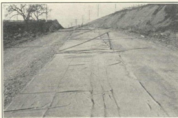
Curing Cement Concrete Pavement on Petaluma-Ignacio Section of Redwood Highway
