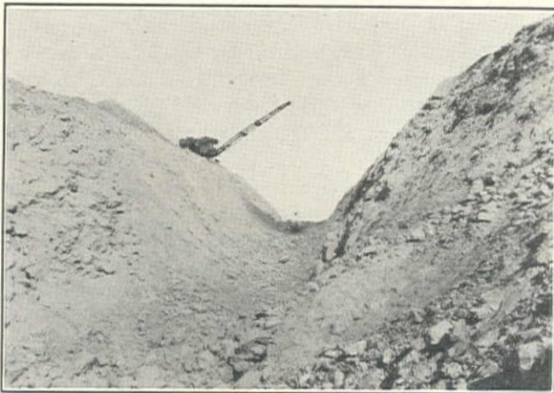
Bucyrus-Erie 50-B Diesel Dragline on 50-ft. Cut at Head of Bully Creek Siphon, Vale Project Main Canal; W. H. Puckett Co. Contractor
