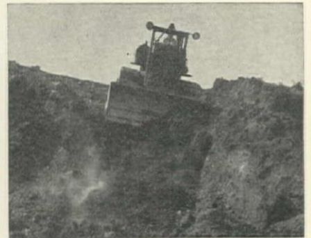
BULL DOZER Leveling Top of Embankment
