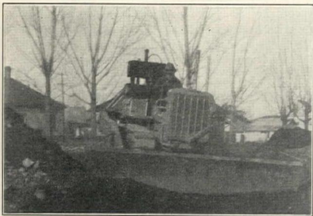
Caterpillar '30' with La Plante-Choate Bulldozer Backfilling 14-ft. Trench on Trunk No. 3, Russell St., Missoula
