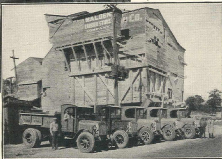
Sterling DC-26, 7 to 8½ tons, a husky, chain drive six
