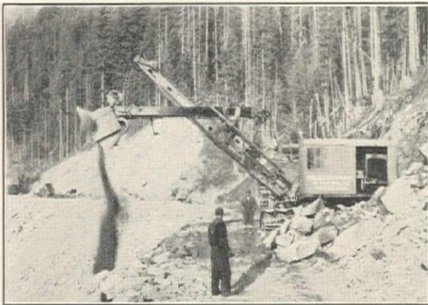
Excavating Trench for Highway Along Shore Line of Lake Keechelus; 1¼-yd. Northwest Shovel in Foreground
