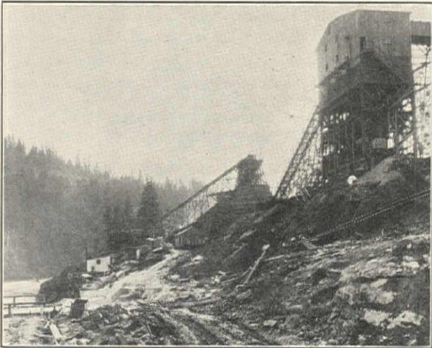
Concrete Aggregates and Mixing Plant Equipped with Tel-smith Crushers and Smith 2-yd. Mixers
