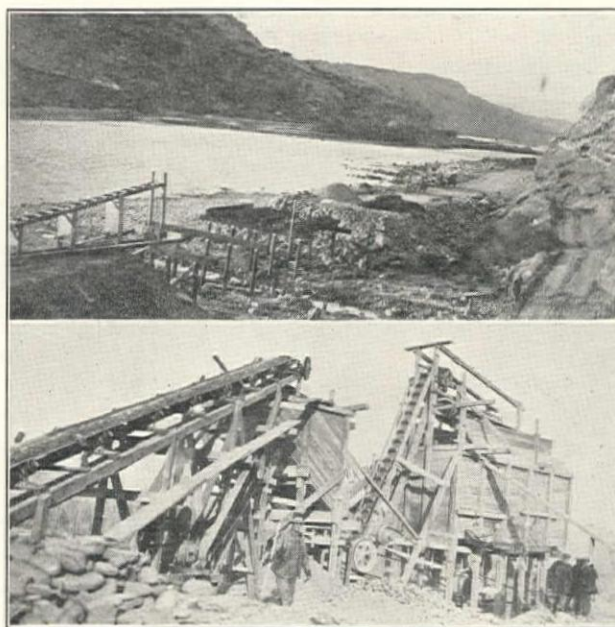
(Upper) Highway Construction in Colorado River Canyon, Looking Upstream from Sta. 400. (Lower) Gravel Crushing Plant Near DeBeque for Surfacing Highway
