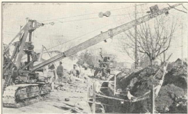
Backfilling Trench on Marin Avenue, North Berkeley, with Austin BF-4 Backfiller. Austin 42-15 Trencher in Distance
