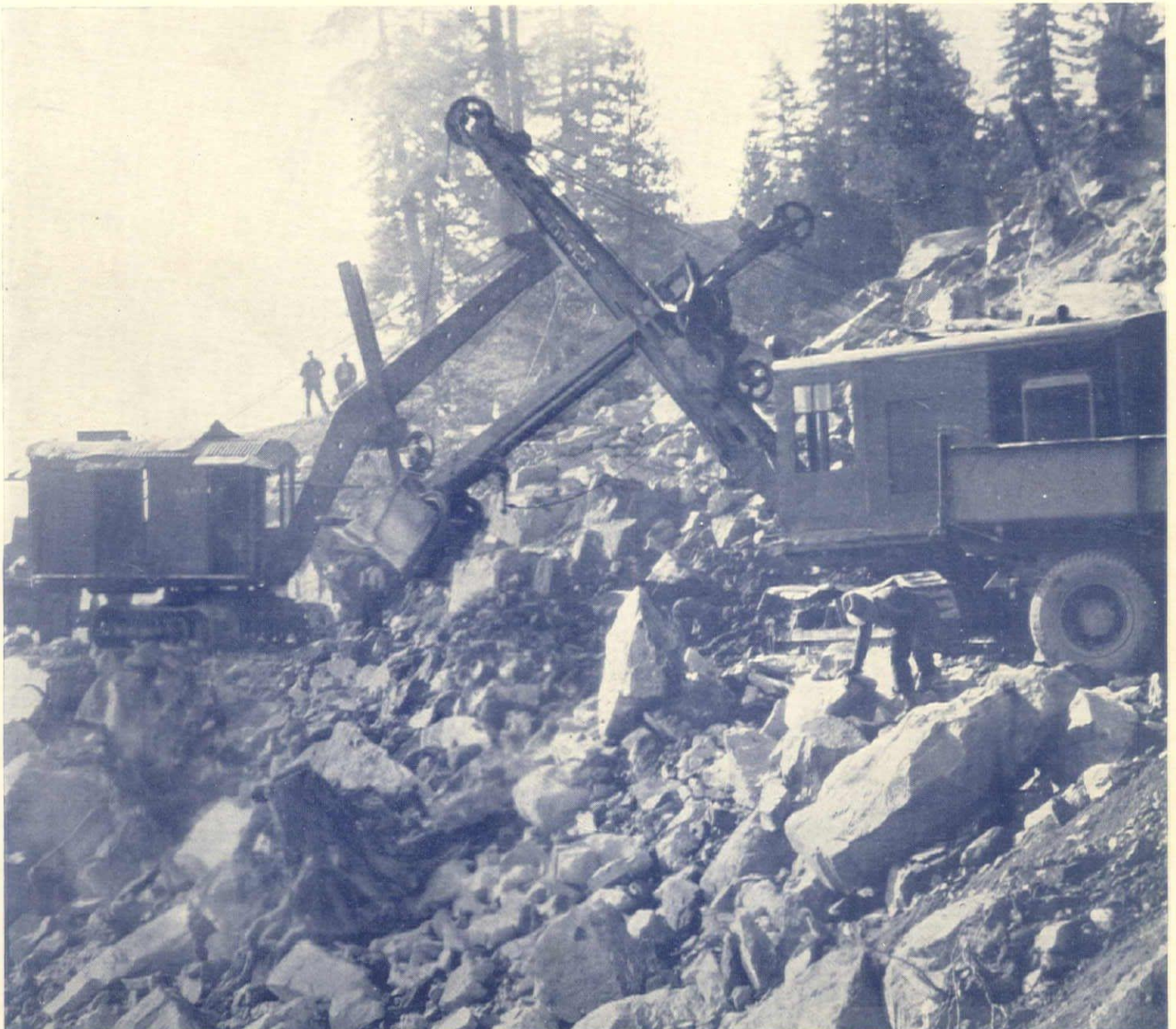
POWER SHOVELS IN SOLID ROCK CUT ALONG THE SHORE OF LAKE KEECHELUS, STATE ROAD No. 2, BETWEEN NORTH BEND AND CLE ELUM, DEPARTMENT OF HIGHWAYS, WASHINGTON; EDWIN J. DUNNIGAN, INC., CONTRACTOR
