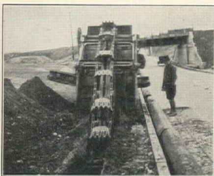
Austin "Little Wonder" Public Service Ditcher—for Sewer, Water, Gas, Oil, and telephone conduit trench excavation. Digs 16 to 38 inches wide and 6, 8, and 10 feet deep
