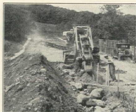
Austin Trench Excavator—the semi-caterpillar machine for deeper and wider cuts. Built in sizes 400, 500, 600, 700, 800, 900.
