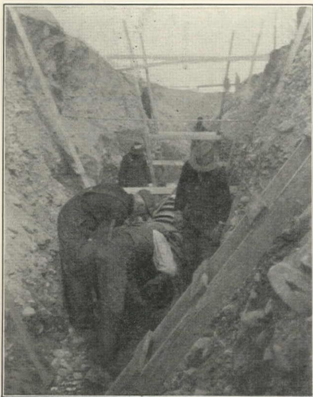
Laying 21-in. Vitrified Clay Pipe on Trunk No. 3 Between Fourth and Fifth St., Missoula, November 28, 1929
