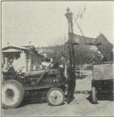
Fordson-Killefer Loader Clearing Street of Excess Material
