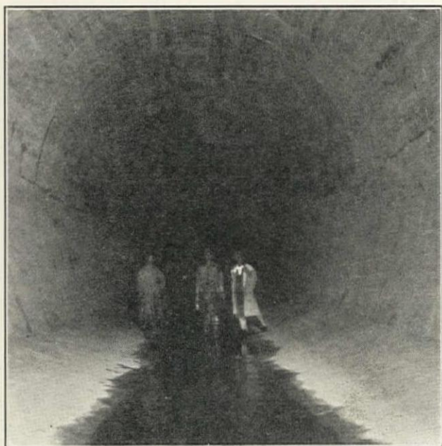
Fig. 9. Finished Section of Horseshoe-Shaped Tunnel 18.5 by 18.5 ft., Maximum Discharge 1750 c.f.s., Between Sand Basin and Regulating Reservoir. Check Valve Emits Ground Water
