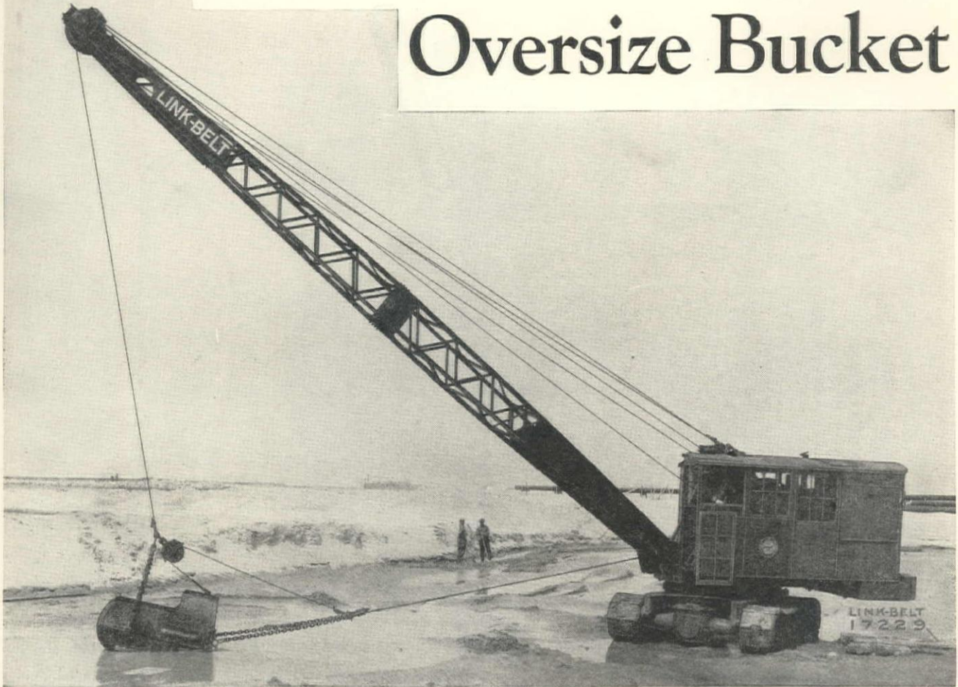
A Link-Belt Dragline with 45 ft. boom and 1 1/4 cu. yd. bucket at work on lake front improvement in Chicago
