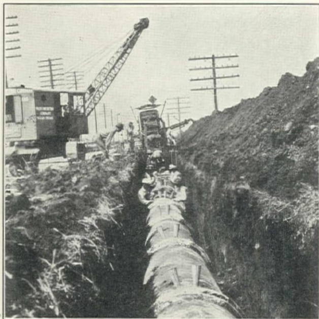
Northwest Power Shovel with Specially Designed Pipe Tongs Lowering 36-in. Cast-Iron Main on Line No. 3, Keating Ave., Dallas. Austin Ditcher in Background. Leadite Joints Being Poured in Fore-ground by Two-Cone Method
