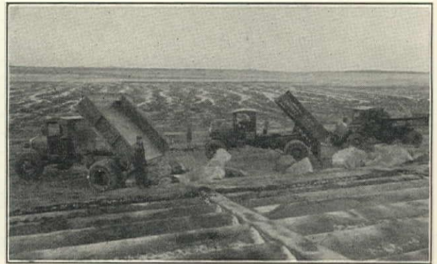
Three Sterling Trucks Placing False Seawall in 8-Ton Loads
