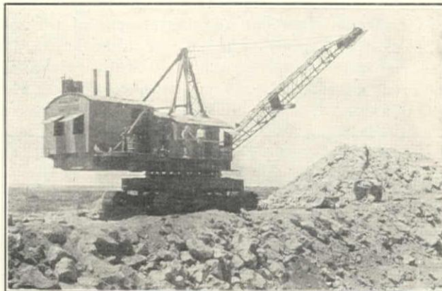
Type 14-B Bucyrus-Erie 3-yd. Diesel-Electric Dragline on Derbon Contract
