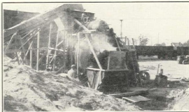
18-Sack Central Mixing Plant on Oswald Bros. Contract for Paving Century Blvd., City of Lynwood, California, Showing Discharge and Loading Hoppers and Loading Pit
