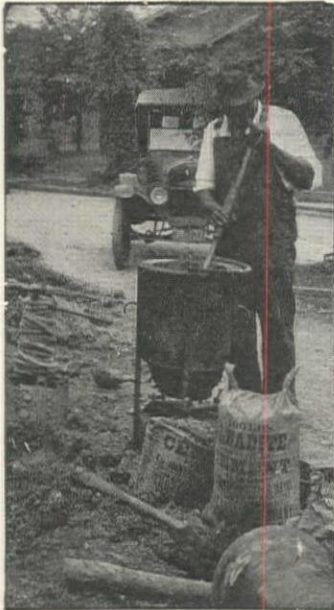
Melting Leadite prior to pouring joint.
