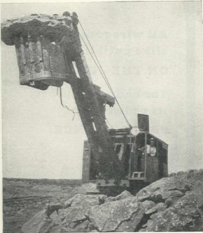
Link-Belt 1¼-yd. Gas Shovel Handling Large Boulder from Quarry of James Stone Co., Richland, Texas
