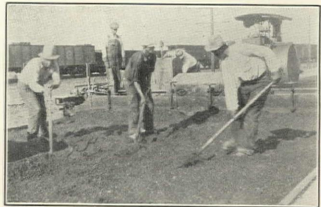
Placing Asphaltic Concrete on Valley Paving & Construction Co. Contract for California Division of Highways, Tulare County
