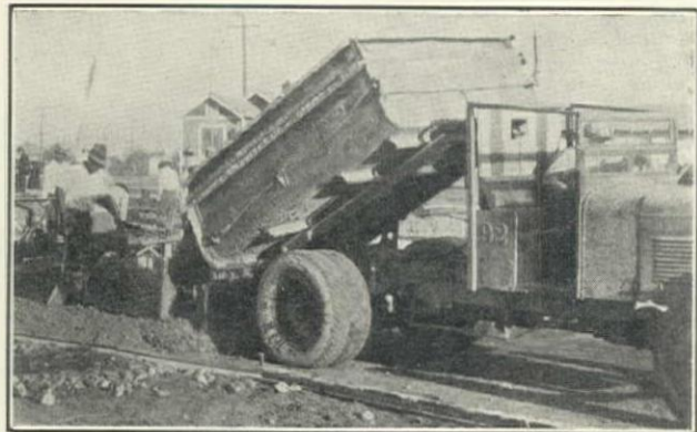
Indiana 5-yd. Truck Dumping Concrete for Century Blvd., City of Lynwood, California, Oswald Bros., Contractors. Lakewood Tamper in Background
