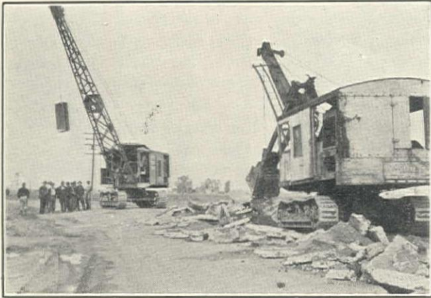
Northwest 1-yd. Power Shovel and Northwest 1-yd. Clamshell Crane on Valley Paving & Construction Co. Contract for California Division of Highways, Tulare County
