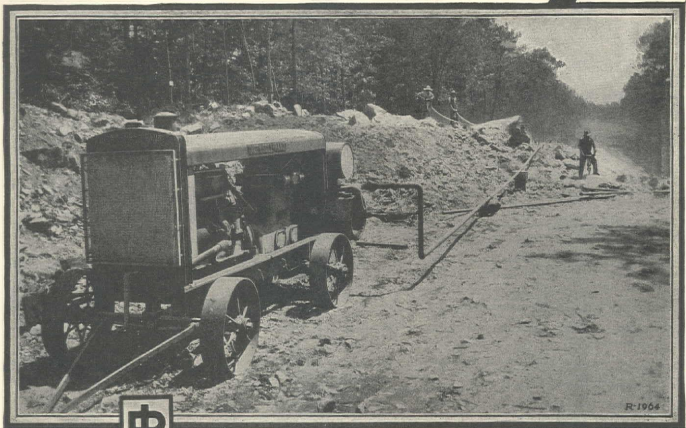
An economical combination—three S-49 "Jackhamers" operating from a single I-R Portable
