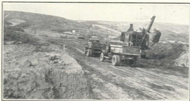
Bucyrus-Erie Power Shovel Loading Into Dump Trucks on County Improvement District 25, Dana Point, Orange County, California, Western Construction Co. Contract
