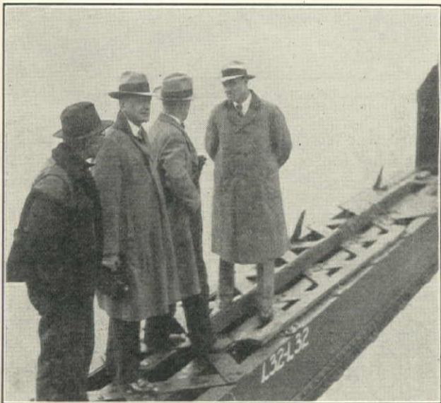
The Final Chord, a 28-ft. Deck Span on the Columbia River-Longview Bridge. Erection of 12,500 Tons Superstructure Steel Completed in 8 Months. Enoch Gerrick, Steel Foreman, in Foreground, and J. H. Pomeroy of J. H. Pomeroy & Co., Erectors, in Background
