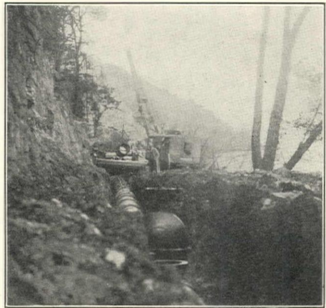
Northwest Power Shovel Laying Cast-Iron Pipe for Lake Waco Aqueduct
