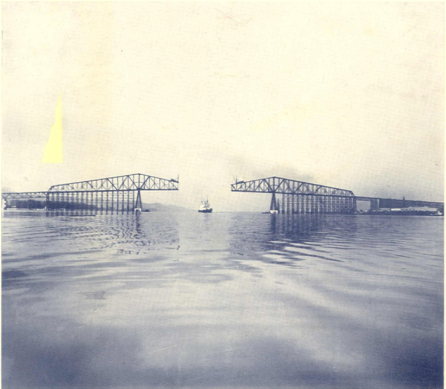
COLUMBIA RIVER-LONGVIEW INTERSTATE TOLL BRIDGE BETWEEN WASHINGTON AND OREGON THREE WEEKS BEFORE COMPLETION OF SUSPENDED SPAN; BETHLEHEM STEEL CO., GENERAL CONTRACTOR; STRAUSS ENGINEERING CO., ENGINEERS
