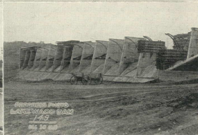
(UPPER LEFT) LORAIN '75' DIGGING CUTOFF TRENCH ALONG CENTER LINE OF DAM. (UPPER RIGHT) NORTHWEST DRAGLINE WITH 60-FT. BOOM PLACING CONCRETE SLOPE PAVING ON LAKE WACO DAM. (LOWER LEFT) CONSTRUCTING SPILLWAY WEIR AND TAINTER GATES. (LOWER RIGHT) SPILLWAY WEIR WITH MOST OF THE PIERS COMPLETED AND TAINTER GATES ERECTED
