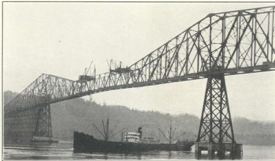
CLOSING SUSPENDED SPAN ON COLUMBIA RIVER-LONGVIEW BRIDGE
