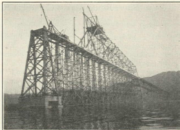
Constructing Anchor Arm on Oregon Side, Columbia River-Longview Bridge, October 22, 1929
