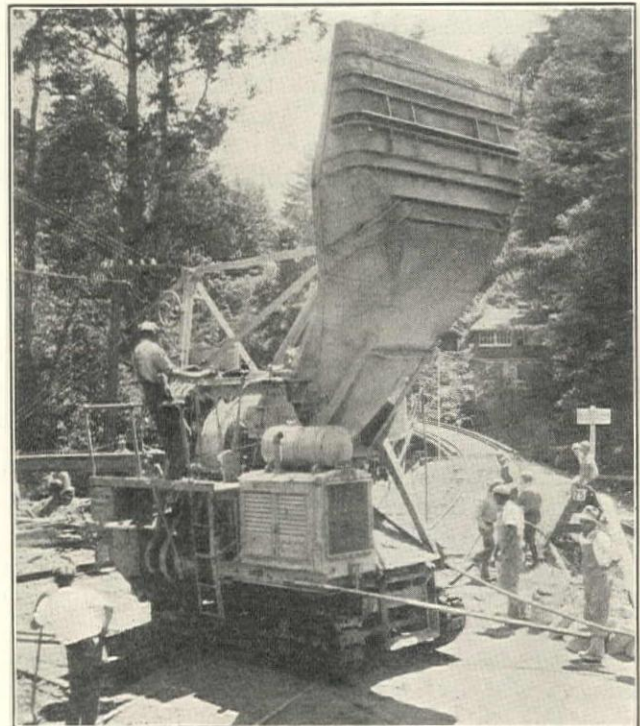
Multifoot 27-E Paver on J. V. Galbraith Contract, Whites Hill-Point Reyes Highway
