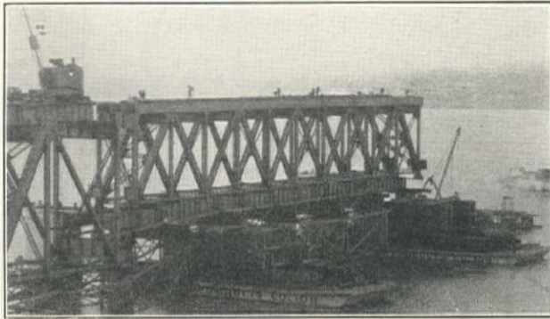
Erecting Deck Span 10 for Suisun Bay Bridge, Industrial Works Locomotive Crane in Left Background, January 22, 1930. Span Floated Into Position on 40 by 125-ft. Barges
