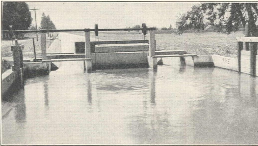
Illustration of Calco Radial Headgate installed on Turlock irrigation project
