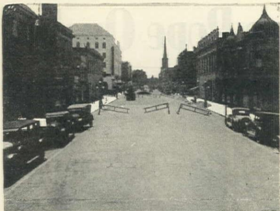
...A portion of Sixth Street between I and L Streets in Sacramento, showing reclaiming work in progress, as well as close up of old, rough pavement.
