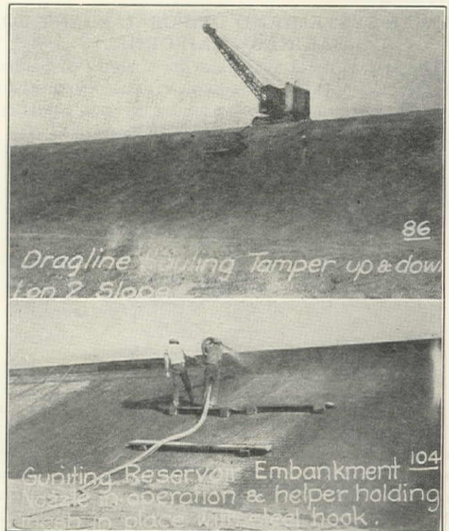
Constructing Chenery Reservoir, Port Costa Development, Calif. H. W. Rohl, Contractor for Embankment Placing and California Gunite Construction Co., Contractor for Lining
