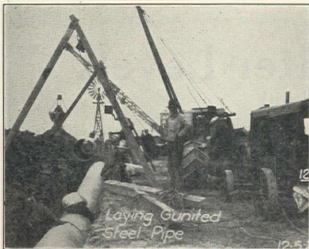
Laying Gunited Steel Pipe on Port Costa Development, Calif., Steel Tank & Pipe Co., Contractors
