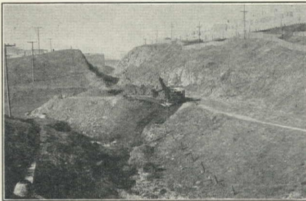
Excavating Trench, Alemany Sewer Section A, Using Osgood Dragline, Clinton Construction Co., Contractors
