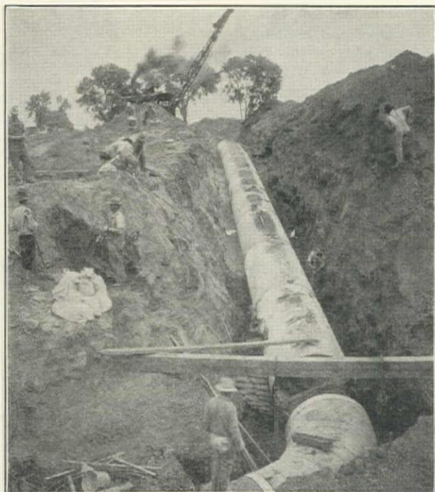
Pipe in Place for Closure Section of 4-ft. Conduit No. 13, City of Denver, Lock-Joint Pipe Co., Contractors
