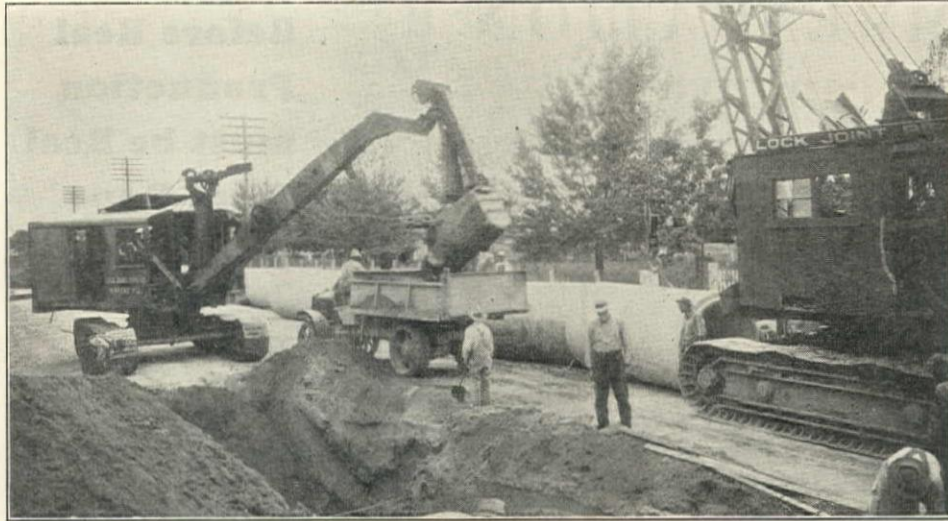
NORTHWEST PULL SHOVEL AND WHITE TRUCK IN USE ON CONDUIT NO. 13, CITY OF DENVER, LOCK JOINT PIPE CO., CONTRACTORS
