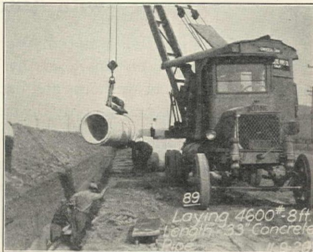
Truck Mounted Universal Crane Laying 33-in. Concrete Pipe (4600 lb. 8 ft. length) Port Costa Development, Calif. American Concrete Pipe Co., Contractors
