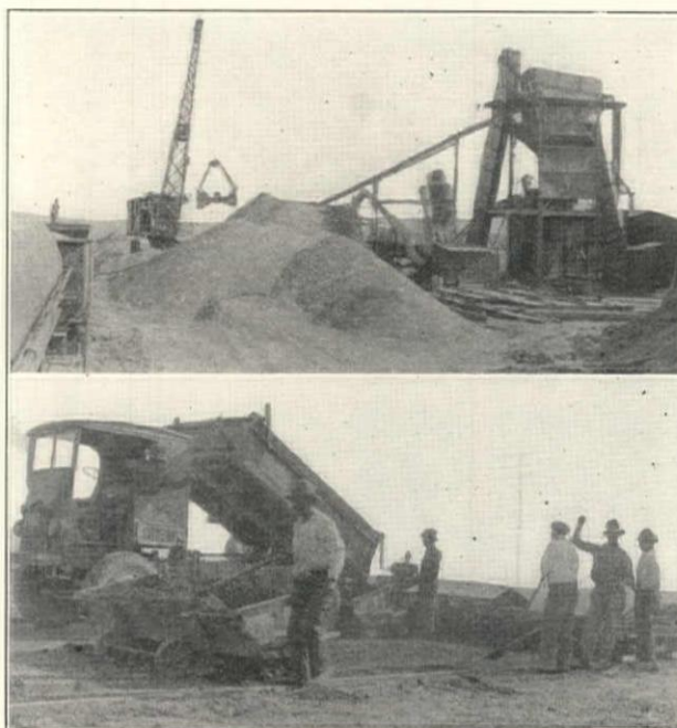
(Upper) General View of Asphalt Plant Showing Northwest 1¼-yd. Clamshell Unloading Stone for Salinas-Chualar Highway Construction. (Lower) Autocar Truck Dumping Asphaltic Concrete Into Spreader Box
