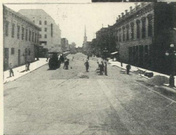
... Another view of the same street during the course of resurfacing. Note disintegrated old surfacing.
