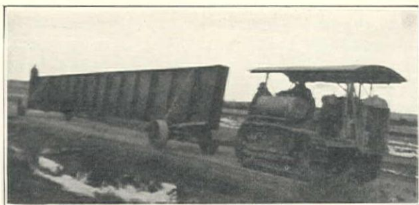
Caterpillar '60' Hauling Steel Girder to Site of Bridge Structure on F.A.P. 277-D
