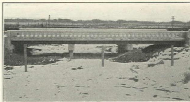
63-ft. Reinforced Concrete Pile Bridge on F.A.P. 277-D
