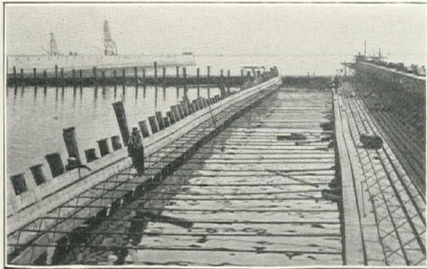
Fig. 2. Outer End of Temporary Creosoted Timber Bulkhead, Long Beach
