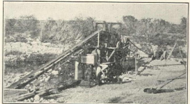
Sand and Gravel Screening and Washing Plant, F.A.P. 132-A
