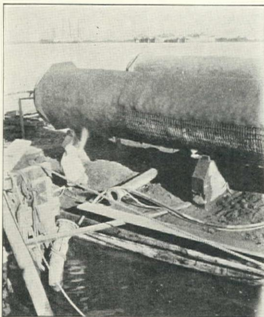
Fig. 4. Gunited Field Sections of 54-in. Steel Pipe on Barge Ready for Submergence
