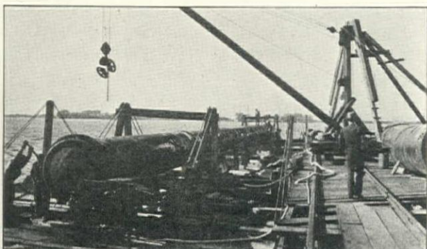
Fig. 3. Field Section of 54-in. Diam. Steel Pipe Ready for Test
