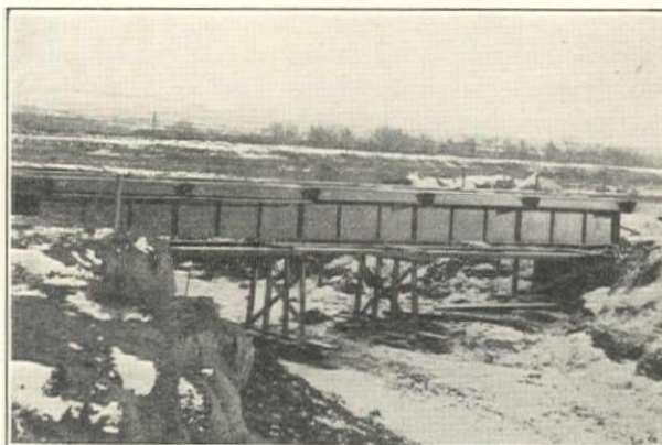
Constructing 140-ft. Steel Girder Bridge on F.A.P. 277-D. Note Temporary Trestle from which Steel is Jacked Into Position
