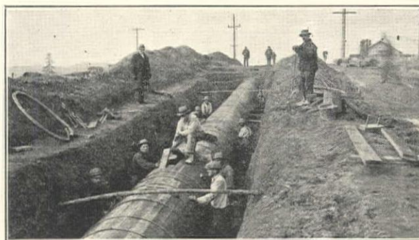
Fig. 13. Reconstructing Cedar River Pipe-Line No. 2 from Reclaimed Staves, Looking North from Near Leo St., Seattle
