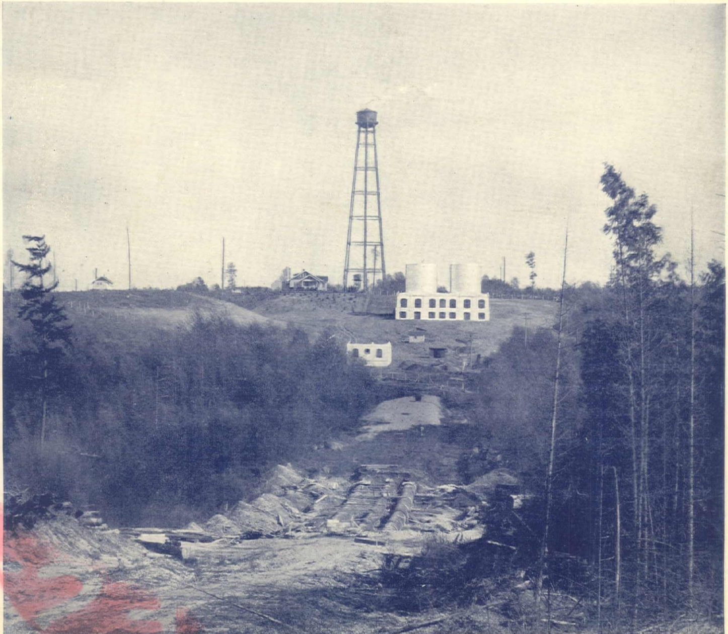
MOLASSES CREEK CONTROL WORKS, SEATTLE WATER SYSTEM. THREE DELIVERY LINES IN FOREGROUND; SMALL CHLORINATOR HOUSE IN CENTER; CONTROL TANKS IN RIGHT BACKGROUND; ELEVATED PRESSURE TANK FOR CHLORINATORS IN CENTER BACKGROUND
