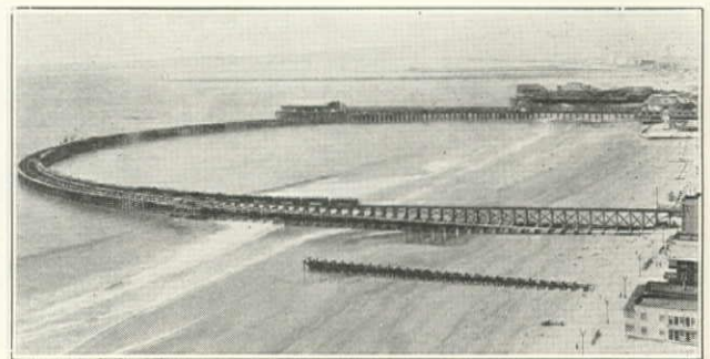
Fig. 3. Substructure for Pier Auditorium Project
