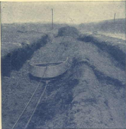
Making a Long Cut-and-Fill
