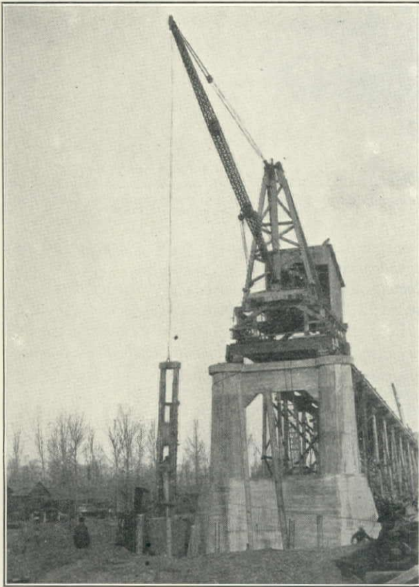
Driving Piling from North River Pier for Falsework Prior to Steel Erection on Missouri River Bridge
