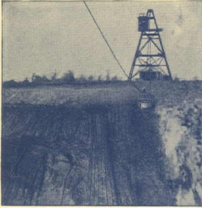
SAUERMAN Scraper with Self-Propelling Head-Tower on Embankment Work
