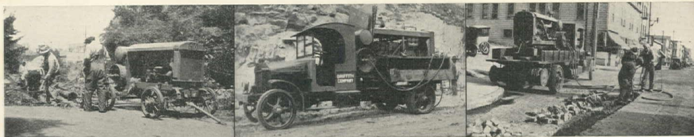
AT LEFT: East Bay Water Company, Oakland, digging pipe ditches with Rix 6. CENTER: One of several Rix sixes operated by Griffith Company, Los Angeles, in road construction. AT RIGHT: Pacific Gas & Electric Co., San Francisco, breaking paving with Rix power.
