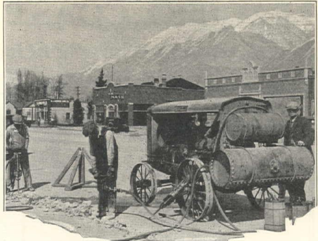
A Sullivan Buster, run by a Sullivan Portable Air Compressor, cutting concrete pavement for lighting conduit, Provo, Utah
