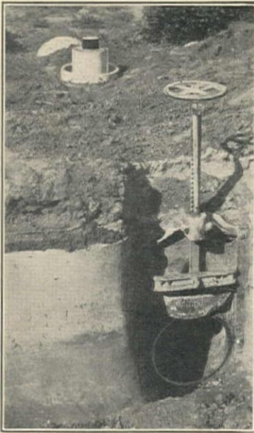
Above: Typical embankment pipe delivery with meter installation.
