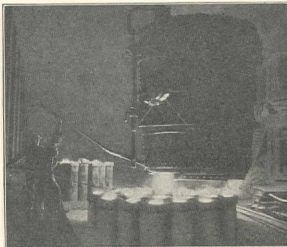
BOTTOM POURING INTO MOLDS
