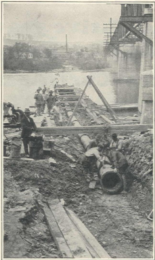
Laying 20-in. c.i. bell and spigot water main across Schuylkill River with LEADITE joints.
