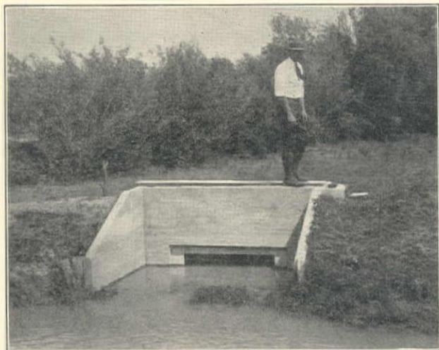
Great Western Meter Installation on 6 sq.ft. Orifice from Main Canal to Large Lateral, Merced Irrigation District
