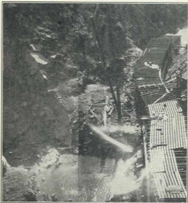
Flume and Excavation for Cushman Dam No. 2, City of Tacoma, L. H. Hoffman, Contractor
