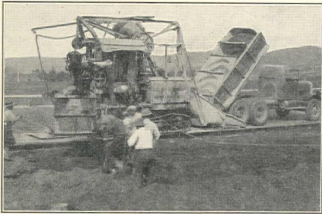
Fageol 6-Wheel, 4-Batch Truck Dumping Into Skip of Koehring 27-E Paver, Eaton & Smith Contract, Junipero Serra Blvd.
