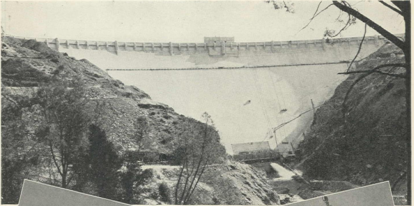
Downstream view of Pardee Dam. Larner-Johnson valves discharging in center foreground.
