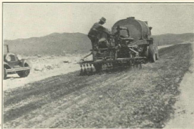
Fig. 1. Distributing Application of Oil Over Gravel Surface
