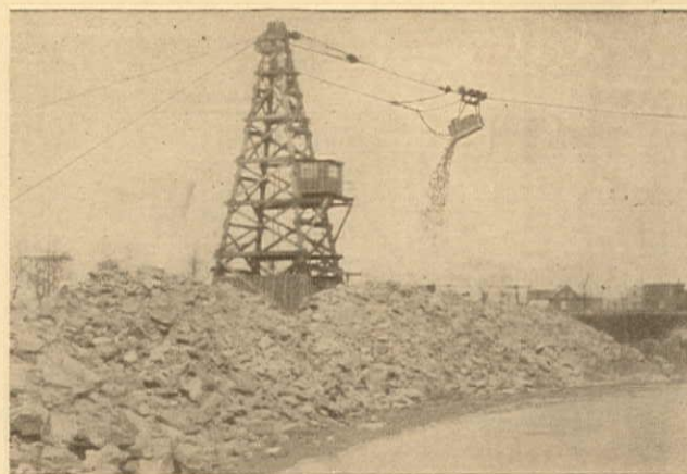
REMOVING BLASTED ROCK FROM CANAL
