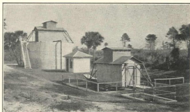
Separate Sludge Digestion Plant for 1.2 M.G.D. Flow and 2-Hour Detention. Clarifier in Foreground is 30-ft. Square and Digester is 30-ft. Diameter and 19 ft. Deep Inside. Vero Beach, Florida
