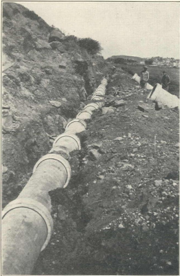
Pumping line to sewage treatment plant, Klamath Falls, Oregon
