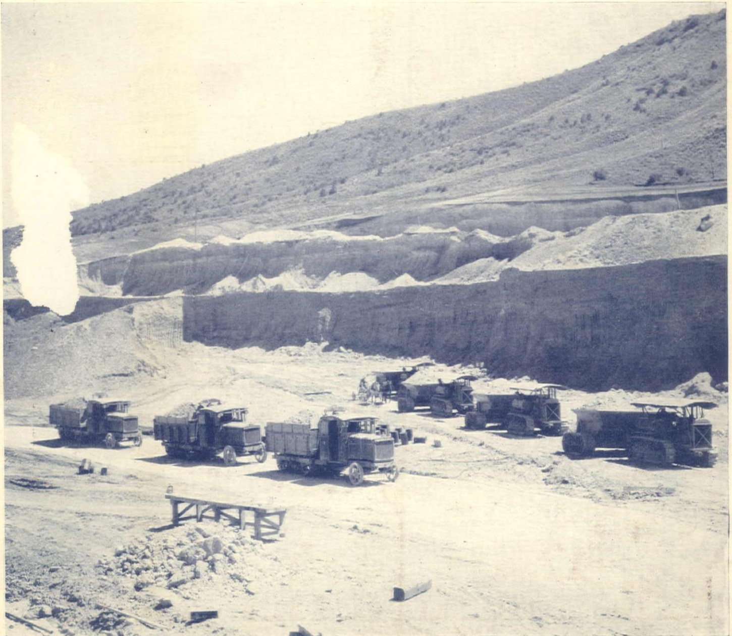
BORROW PIT FOR ECHO ROLLED EARTH-FILL DAM, SALT LAKE BASIN PROJECT, BUREAU OF RECLAMATION, UTAH
