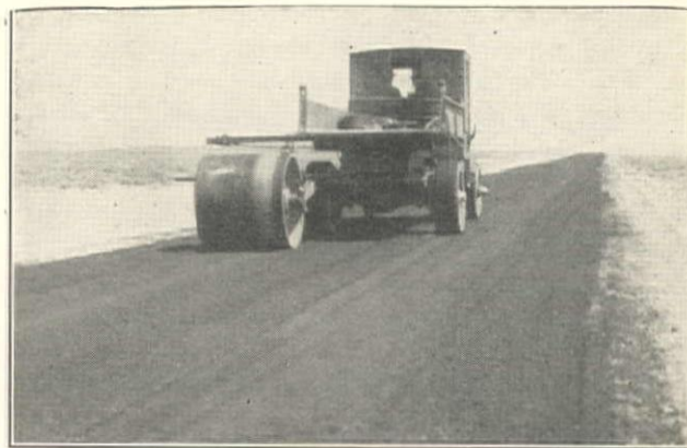
Fig. 3. Compacting Shoulders with Light Roller Where Traffic Holds to Center of Road
