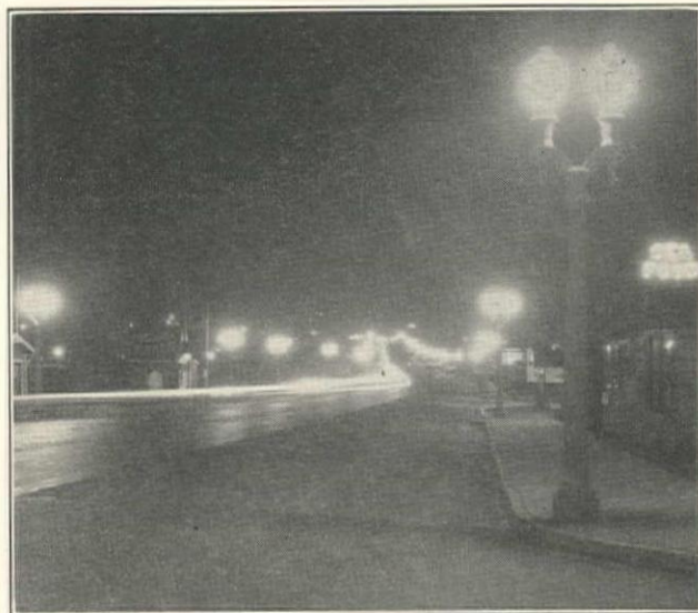
Fig. 3. Night Illumination in Pismo Beach Using Marbelite Double Light Standards and Prizmalite Glassware with 250-c.p. Lamps
