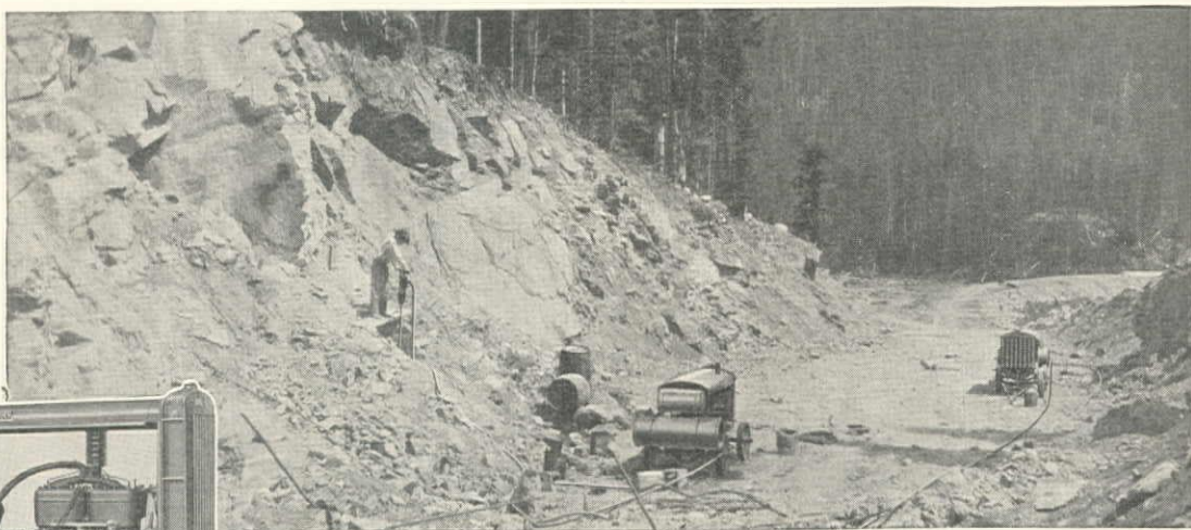
Two of the 23 Sullivan Vibrationless Compressors at work in Snoqualmie Pass. At left, Sullivan 310-ft. Vibrationless Compressor, on steel wheels.
