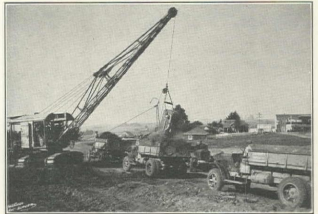
White Trucks and P&H Dragline on E. C. Coats Contract from Loleta to Beatrice, Humboldt County, for California Division of Highways
