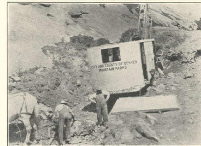
Osgood Gas Shovel Excavating Highway
