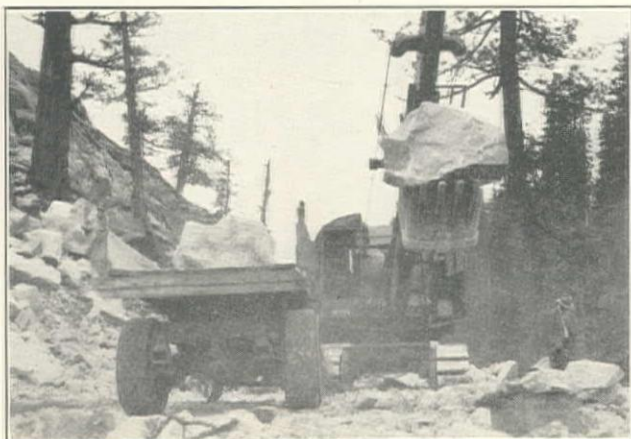
P&H 206 Shovel on T. E. Connelly Contract, Nevada and Placer Counties, for California Division of Highways
