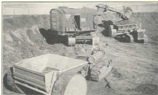
Bucyrus Erie 50 B Shovel, Equipped with 100 hp. Atlas Diesel Engine, Loading Le Tourneau 16-yd. Dump Carts, North Approach to Southern Pacific R.R. Bridge Over Suisun Bay, R. G. Le Tourneau, Contractor
