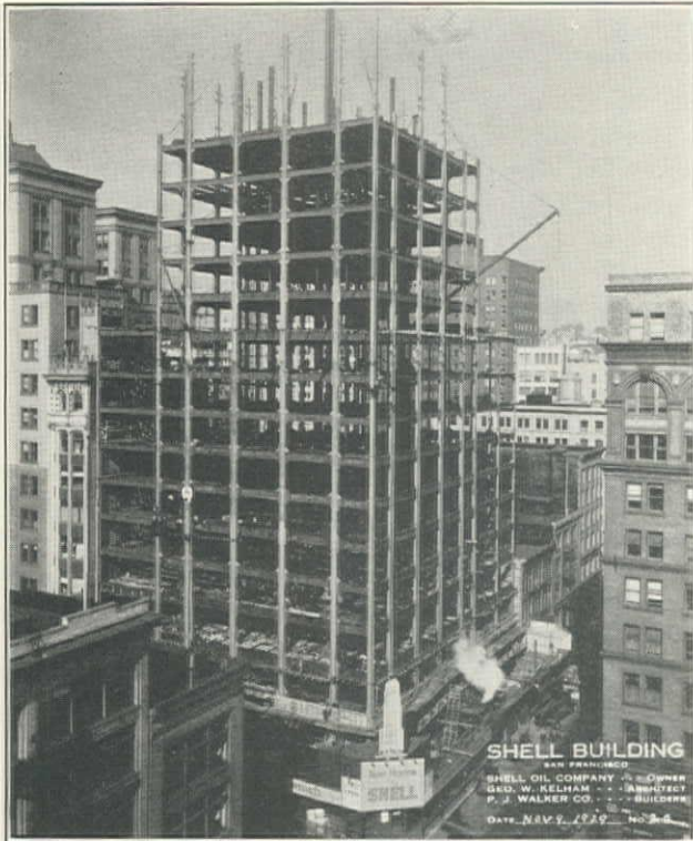
Fig. 1. Erecting Structural Steel Frame for Shell Bdg. November, 1929. Architectural Perspective of Building Shown on Sign at Corner of Bush and Battery St.
