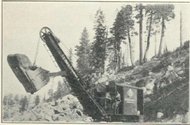
Lima '101' Ohio Power Shovel on T. E. Connolly Contract in Nevada and Placer Counties for California Division of Highways
