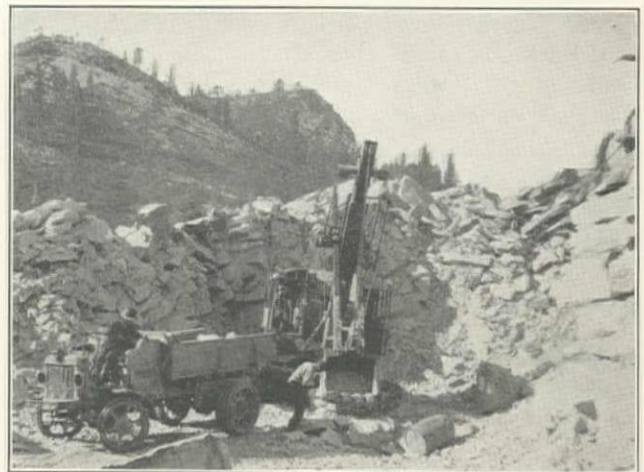
P&H Shovel and Autocar Truck in Granite Cut, Strawberry Phillips Section of Placerville-Tahoe Highway, El Dorado County, California, for Bureau of Public Roads, Nate Lovelace, Contractor
