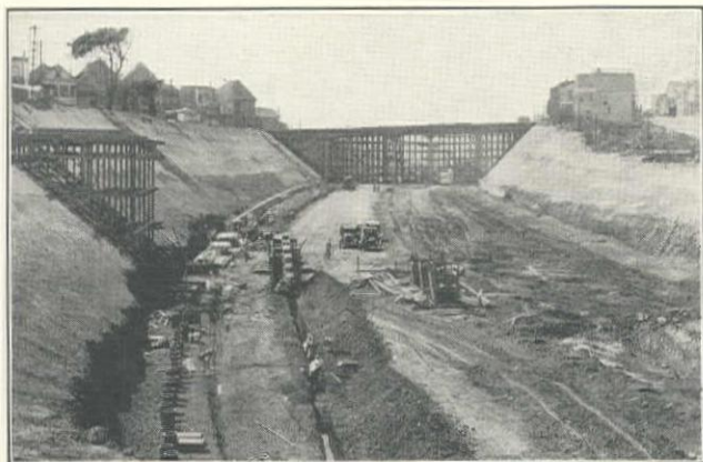
Constructing Bernal Cut Project for City and County of San Francisco, MacDonald & Kahn, Contractors, Showing Austin Trencher in Operation
