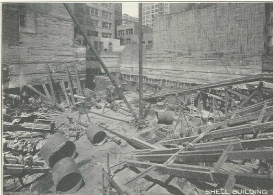
FIG. 2. PREPARING FOUNDATION ON AUGUST 10, 1929. EXCAVATION IN PROGRESS IN LEFT FOREGROUND, SHELL SECTIONS FOR CAISSON BEING STORED NEAR HOLE. TRUCKING INCLINE IS IN RIGHT BACKGROUND
