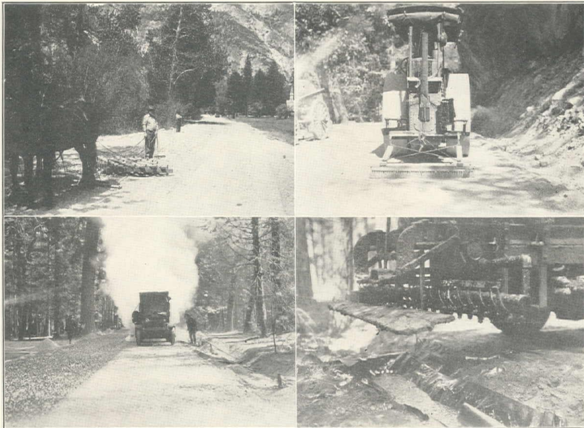
Fig. 1. (Upper Left) Use of Harrow to Shake Down Filler to Bottom of Base Course on Asphaltic Penetration Macadam, Yosemite Valley Highway. (Upper Right) Brooming Screenings Into Voids and Rolling in One Operation. (Lower Left) Applying First Coat of Asphalt to Second Half of Road. (Lower Right) Bleeding Truck to Insure That All Sprays Are Clean Before Spreading Asphalt on Road. These Tar Paper Troughs Will Later Be Collected and Burned
