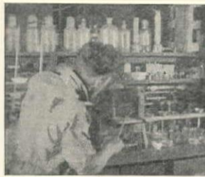
Left — Analyzing the iron for percentages of carbon, silicon, phosphorus, manganese and sulphur
