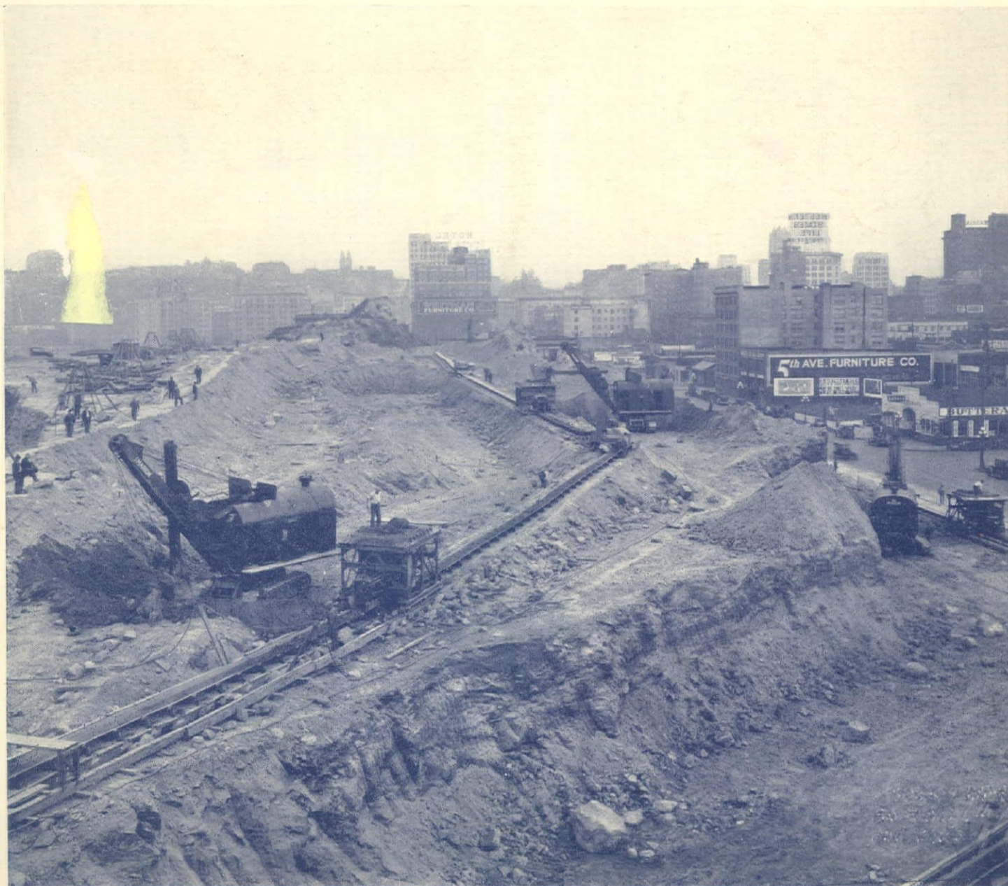
DENNY HILL REGRADE No. 2, SEATTLE. A 4,000,000-CU.YD. EXCAVATION PROJECT HANDLED IN A UNIQUE MANNER
