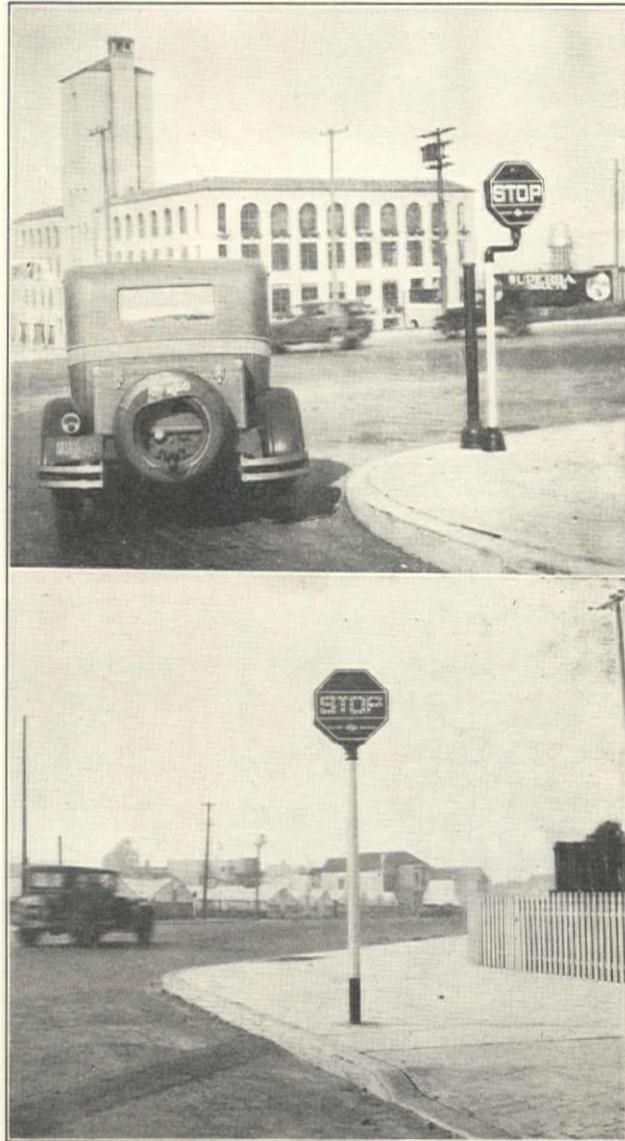
Fig. 2. (Upper) Wired Stop Sign at Intersection of Bayshore Blvd. and Ware St. Pipe to Left of Arterial 'Stop' Will Carry Automatic Signal. (Lower) Battery-Operated 'Stop' Sign at Intersection of Bayshore Blvd. and Faith St.
