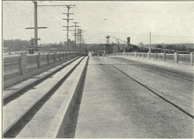
Denver Ave. Viaduct Showing Roadway, Car Track, Special Traffic Strip, Curb, and Handrail Details
