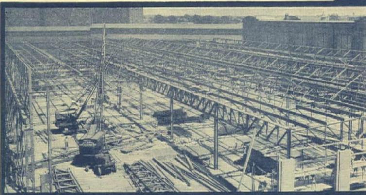
Steel for this type of building is easily erected with these two Universals. 1400 tons were set in 25 crane days.
