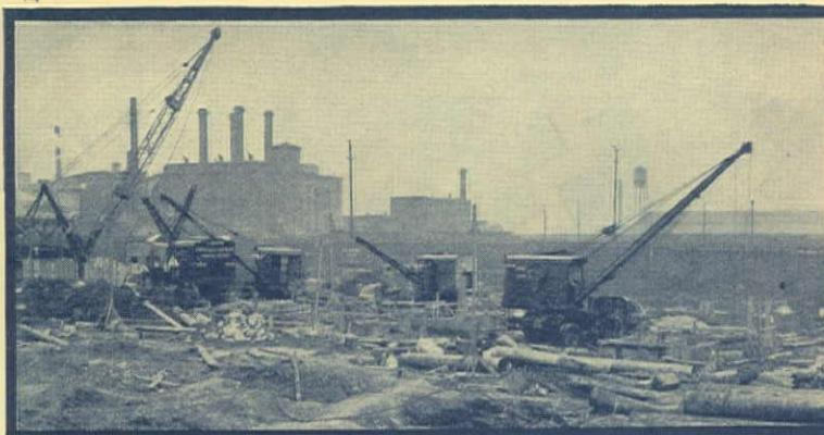
Universal Truck Cranes operating with skip boxes, digging 30 ft. pier holes on the \$10,000,000 Pennsylvania Warehouse, Jersey City.
