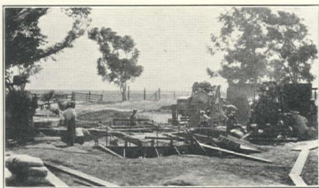
Placing Reinforced Concrete Foundation for New Pittsburg Standpipe
