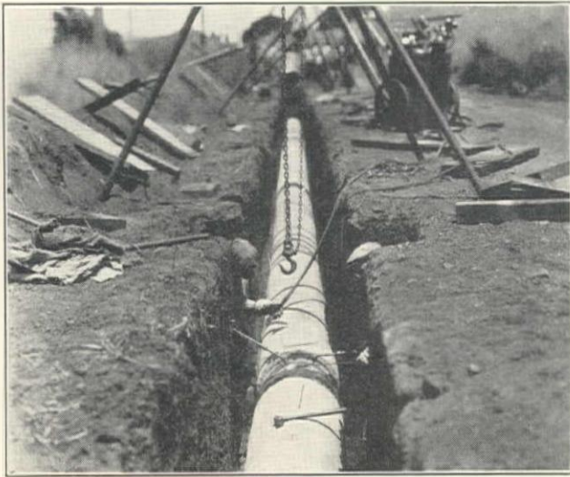
Welding Sections of 30-in. Steel Pipe, Gunite Covered
