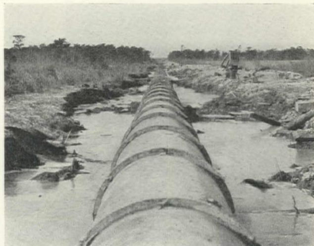
Fig. 6. Section of a Completed 60-in. Cast-Iron Supply Line Laid on Slight Grade Through Marsh Land
