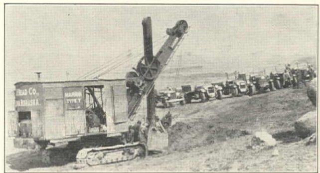
Marion Shovel and White Trucks on North Crow Dam for City of Cheyenne, Wyoming. A. H. Read Co., Contractors
