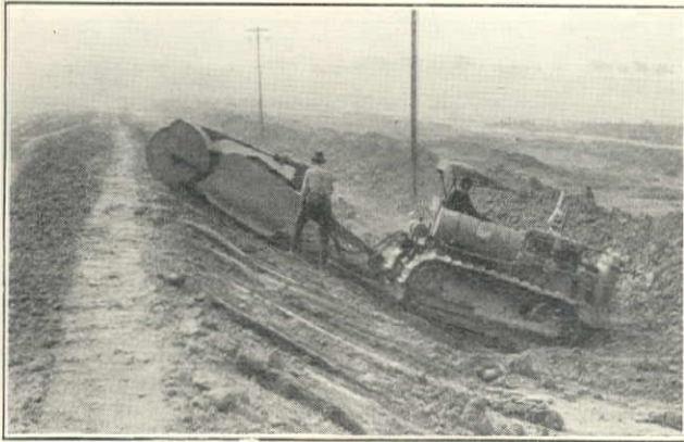
Rough Trimming Embankment Slopes on Chenery Reservoir, Port Costa Development, H. W. Rohl Co., Contractors
