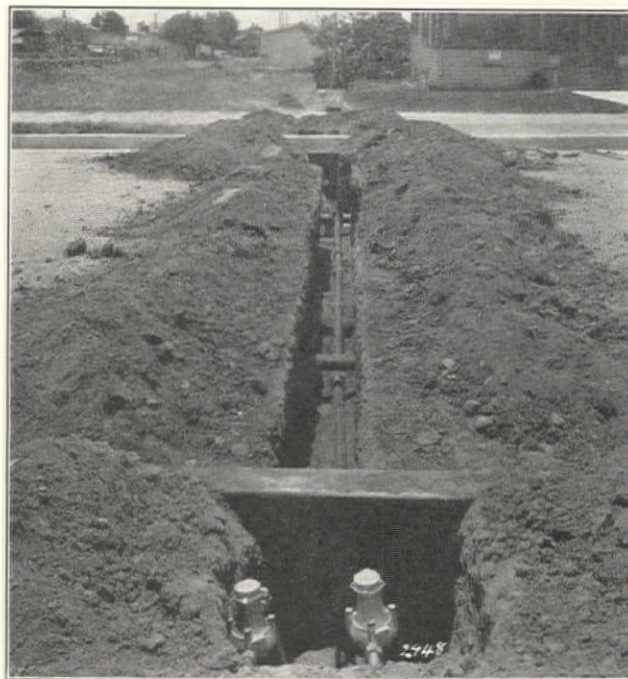
Laying 2-in. Cast-Iron Water Service in a Street in Los Angeles, Feeding Two Lots Through \frac{3}{4} -in. Trident Metered Services
