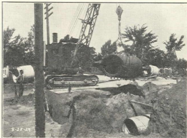
Lowering 54-in. Rensselaer Valve Into Trench, Conduit No. 13 for City of Denver, Colorado, Lock-Joint Pipe Co., Contractors
