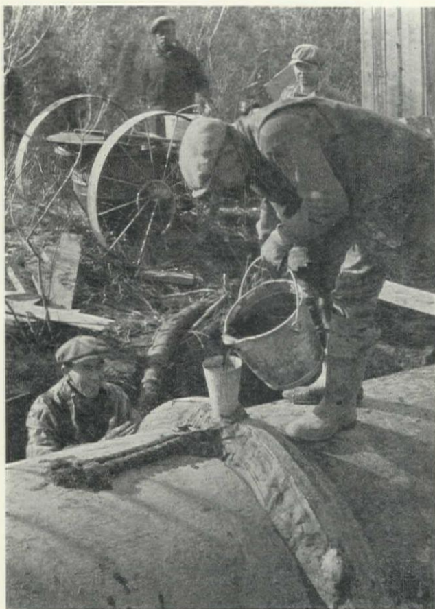
Fig. 5. Pouring a Joint on a 60-in. Cast-Iron Supply Line
