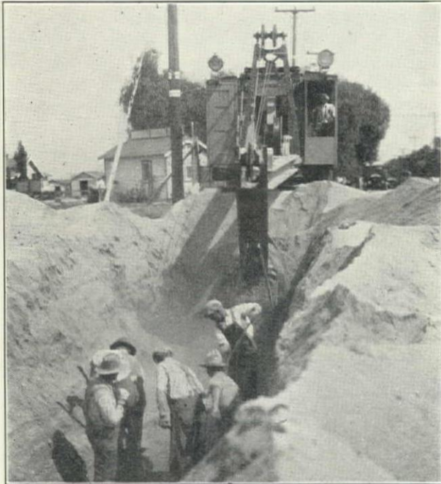
Constructing Hume Reinforced Concrete Van Owen Avenue Pipe-Line for City of Los Angeles, Using Link-Belt Trench Hoe Excavator, American Concrete Pipe Co., Contractors
