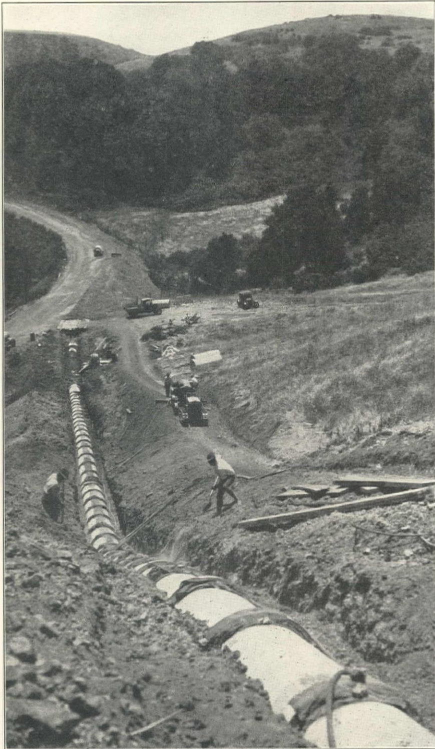
Moraga Aqueduct, East Bay Municipal Utility District, Oakland, California. 8800 feet of 30 and 36-in. Hume Pipe, 25 to 115-ft. head.
