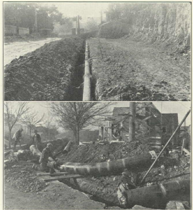
(Upper) Lowering Cast-Iron Water Main Under Pressure as Street Grade Is Cut Down. (Lower) Welding Steel Pipe to Fit Curved Trench in Berkeley
