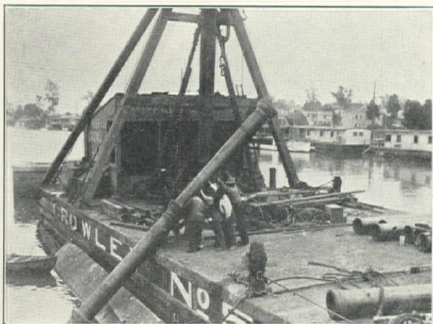
Laying 12-in. 'Ward Joint' Cast-Iron Pipe Main Across Alameda Estuary Between Oakland and Alameda
