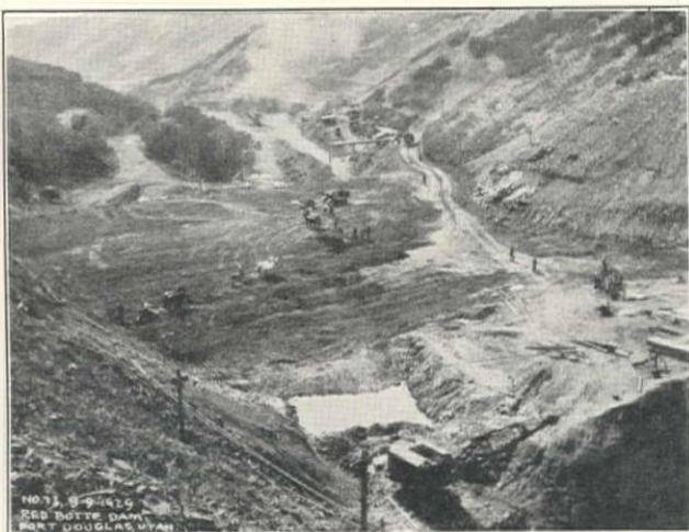
Utah Construction Co. Placing Earth Embankment in Red Butte Dam, Utah. Cutoff Trench Excavation in Progress in Lower Right Background
