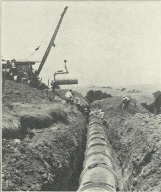
Laying 36-in. Reinforced Concrete Pipe on Schedule 2A, Moraga Aqueduct, East Bay Municipal Utility District, Bent Concrete Pipe Co., Contractors (Now American Concrete Pipe Co.)
