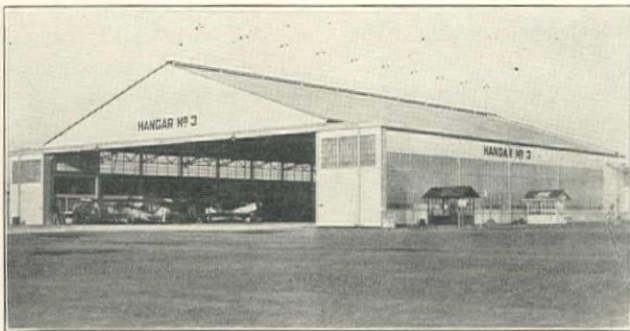
Steel Frame and Corrugated Iron Hangar Construction at the Oakland Municipal Airport
