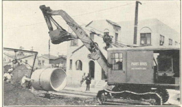
Northwest Pull Shovel Placing 54-in. Concrete Pipe on Unit No. 2 of Berkeley Storm Drain System, Fredrickson & Watson Construction Co., Contractor
