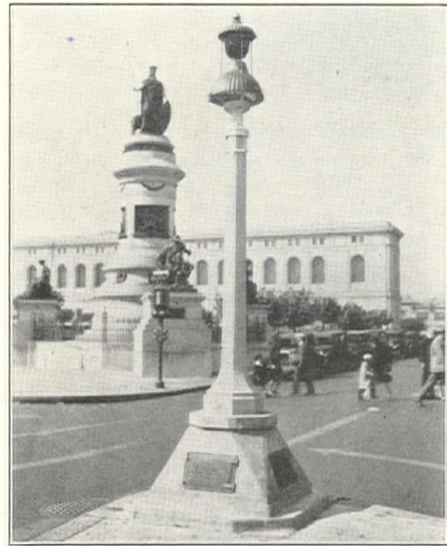
Fig. 9. Detail of Vehicular Warning Beacon on Safety Island at Intersection of Market, Eigheh, Grove, and Hyde St. Control Boxes House Meter, Switch, Fuses, Flasher, and Relay to Street Lighting Circuit. Combination Traffic Signal, Pedestrian Signal, and Street Name Sign in Background by Statue
