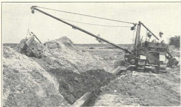
W-K-M Swinging Boom Equipment Used with Caterpillar Tractor for Backfilling Trench
