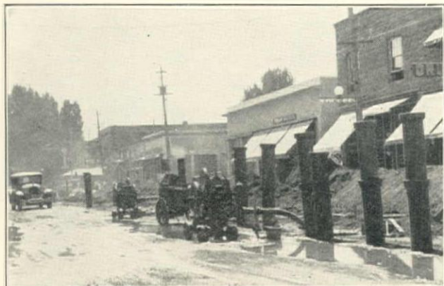
Constructing Alturas Sanitary Sewer, Heafey-Moore Co., Contractor. Barnes Diaphragm Pump in Center Background
