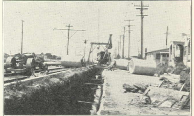
Rocca & Caletti Laying 54-in. Hume Pipe on Sacramento St., Berkeley Storm Drain System, Unit No. 1. Gantry Crane and Northwest Shovel in Background
