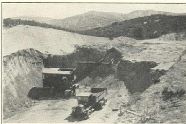
Northwest 1\frac{1}{4} -yd. Gas Shovel Loading Into Truck on Nevada Contracting Co. Job, S.D.-12-F, San Diego County
