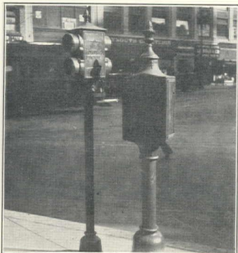
Fig. 4. Pedestrian Signal on Left and Control Box for Intersection on Right
