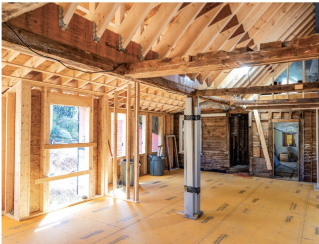
The new vaulted-ceilinged, one-story ell connects the oldest part of the house (in the back of the space) to the two-story addition. The antique timbers salvaged from the old ell will be a dramatic interior element that also provides some support.
