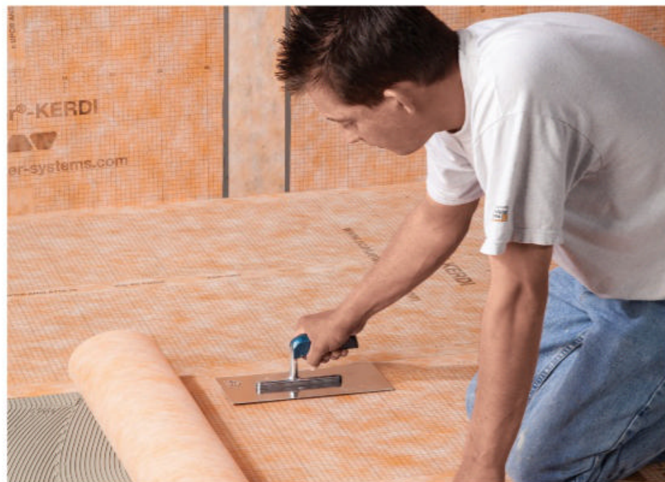
Sheets of Kerdi waterproof membrane (schluter.com) install over thinset mortar, then are covered with more thinset to receive tile. Strips applied at seams and floor and wall joints ensure a waterproof seal.
