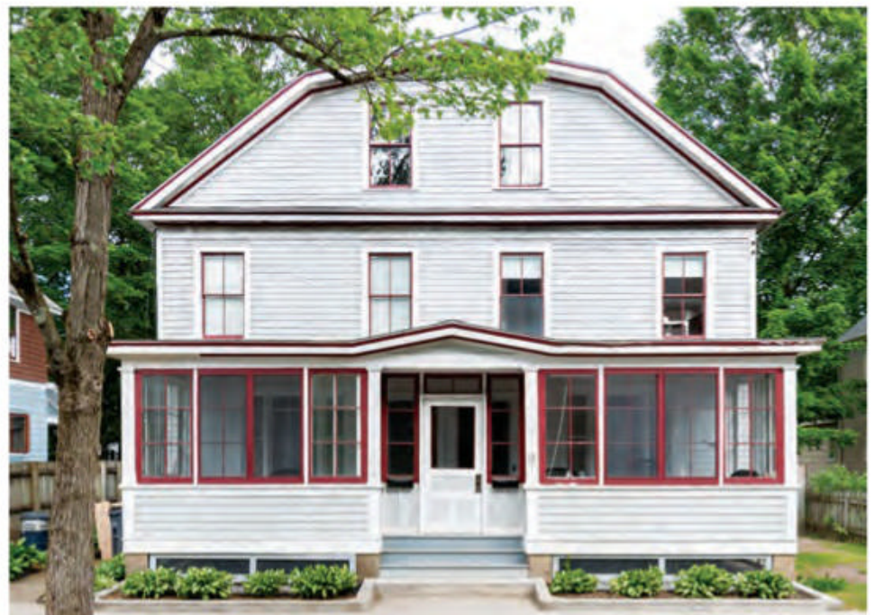
HOMEOWNERS, HOUSE BEFORE: MEG REINHARDT
