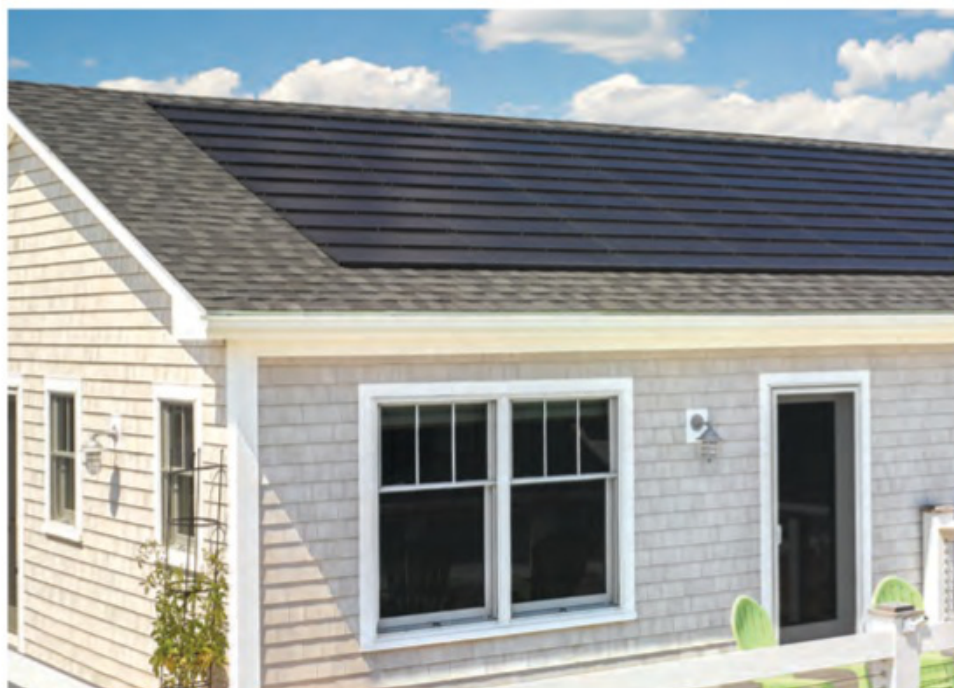
Solar roof shingles, such as these from CertainTeed, are less obtrusive than PV panels.
