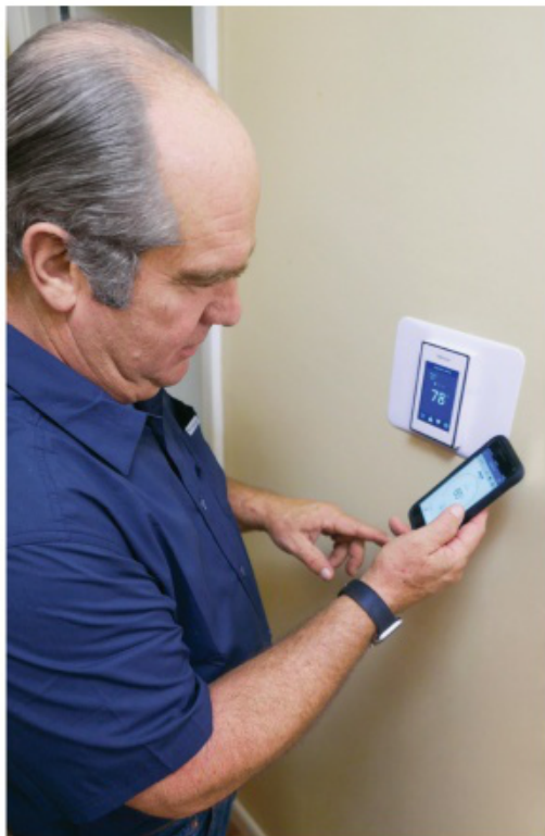
Richard Trethewey sets up a smartphone to communicate with the Invita 564 WiFi thermostat, which operates on just two wires.
