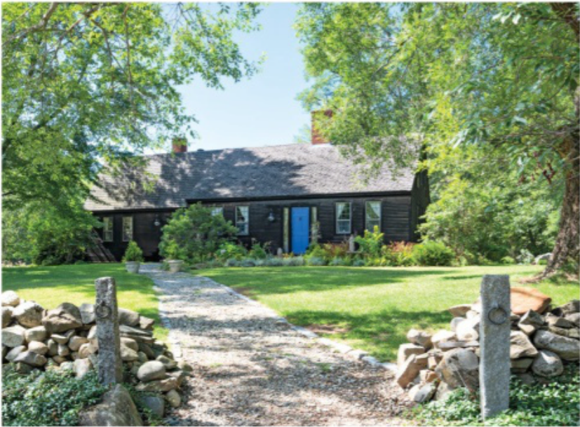
BELOW: The house's vinyl siding was replaced with low-maintenance quartersawn pine clapboards stained with a mix of linseed oil and turpentine and weathered to a nearly black gray.
