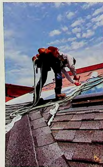
Shown: For a durable, long-lasting roof, crews installed WeatherWatch® Mineral-Surfaced Leak Barrier beneath Timberline Ultra HD Shingles.
