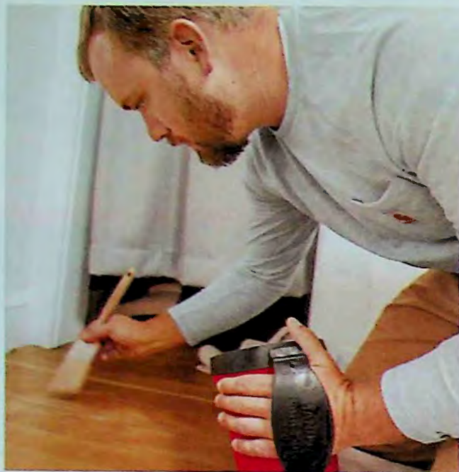
After sanding out the damaged floor finish, Nathan Gilbert protects the wood with a water-based polyurethane.
