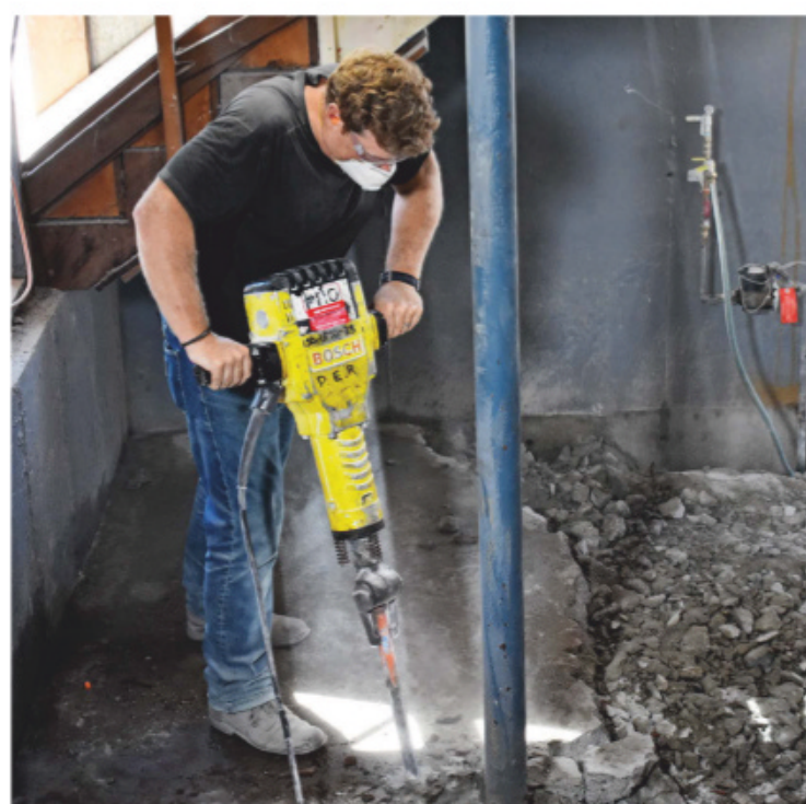
RIGHT BOTTOM: Kevin O’Connor jackhammers the existing basement floor to gain headroom for finished spaces on the lower level.
