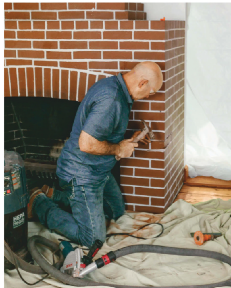
Mason Mark McCullough replaces a damaged brick in a fireplace surround. Changes to stone or marble can also indicate potential trouble.
