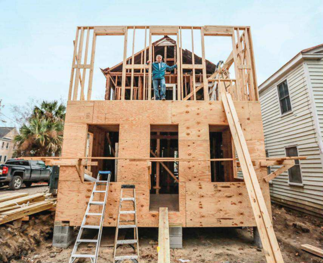
ABOVE: Tom Silva checks out the framing on the two-story addition, which will hold a guest room on the ground level and a master suite above it.
