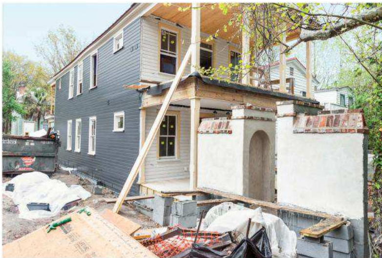
ABOVE: Tom Silva checks out the framing on the two-story addition, which will hold a guest room on the ground level and a master suite above it.
