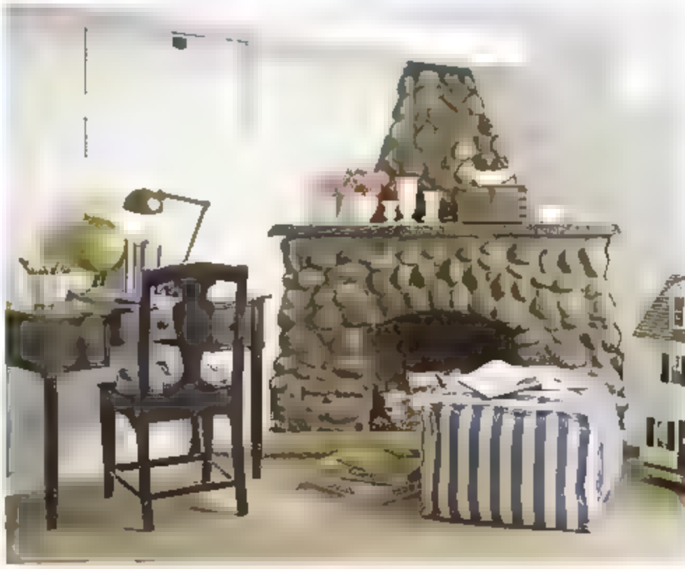
The river stone fireplace built by Mark's father and grandfather finally has a worthy setting, with V-groove pine-paneled walls. The pull-down door high up on the wall accesses a crawl space.
