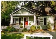
BEFORE: This Daguerre-era cottage was hiding its woods in a quiet 19th-century neighborhood.
