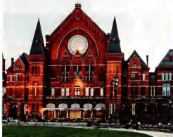
ABOVE: Landmarks include MUSEUM the 1870 home of the Czechs' Synagogue and the Carlsberg Brewery. A large portion of Over the Rhine is on the National Register of Historic Places.
