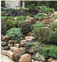
A "living" wall of boulders and plants is a handsome alternative to a rot-prone retaining wall made of landscape timbers.
