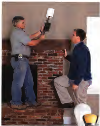
ABOVE: TOH general contractor Tim Silva places a wall sconce above the fireplace in the new family room. "We're using CFLs in these fixtures," says homeowner Joe Tilius. RIGHT: New bulbs that meet the stricter energy standards have been introduced in the past couple of years. Including the SuperSaver halogen bulb (left) from Sylvania and the Ambient LED (right) from Philips.
