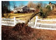
Damaged fence posts can be restored safely by installing some leverage, either with a hydraulic bottle jack or a long 2x6.
