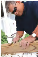
Holding a rail with its level facing up, Tom Silva smooths the bottom of a dovetail notch in a 4x4 post. A dovetail notch could compromise the post's strength.
