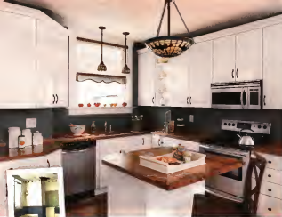
BEFORE: The dreary kitchen was cramped and poorly laid out. AFTER: Nine walls, including mahogany stone-clad fireplace, black counters, and stainless-steel appliances, all installed by the homeowner, help bring a lighter, brighter feel to the space.
