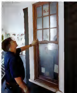
Tom Silva examines a newly installed double replacement window. It looks like the original but has insulated glass and tight weatherstripping.
