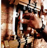
AFTER: Leaving PEX tubing along a wall in a subfloor. Richard will push one end to the manifold's return side. A three-foot 1/2-inch return cut is a convenient way to the manifold to keep the water flow in that area.
