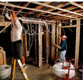
ABOVE: Richard leads the PEX tubing to heating contractor Aron Perry who pushes it using a joint borer. A single length of tubing will loop around each first-floor room. RIGHT: Perry uses a rubber mallet to tap the PEX into the aluminum trays. By evening out the tubes using his compressor, he ensures a balanced panel transfer
