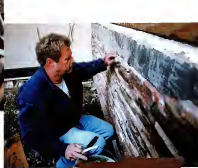
ABOVE: JCM Masonry continues Roger Cook's specialty finesse on a series of natural stone veneer to continue his running pattern on the foundation wall. He leaves his tools and materials close at hand. COURTESY FROM LEFT: Specialty cut pieces fit outside corners, a pointing trowel adds finish touch, and masonry mortar for the backing the back of the stone, and a large bag of dry-lime plaster to keep the surface random and varied.
