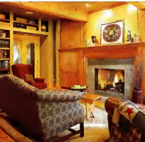
ABOVE Though the original design called for a masonry fireplace and an exterior stone chimney, the homeowners saved $20,000 by using a composite surround and a deep-in-fabric that vents through the roof.
