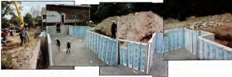
A crew from Superior Walls installs the foundation—panels of insulated concrete that are set on a bed of crushed stone, adhered to each other with a urethane adhesive, and then bolted together. The entire foundation was built in a day, no curing time needed.
