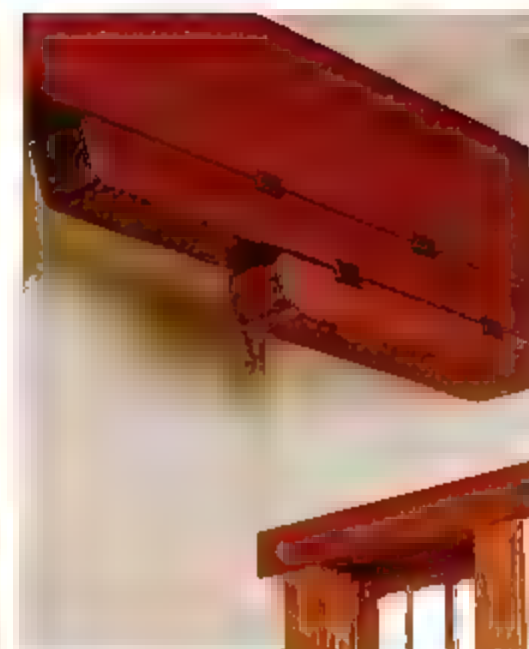
The elegant bracketed ceiling beams are in fact structural, made of engineered wood boxed in mahogany. They support the second floor.
