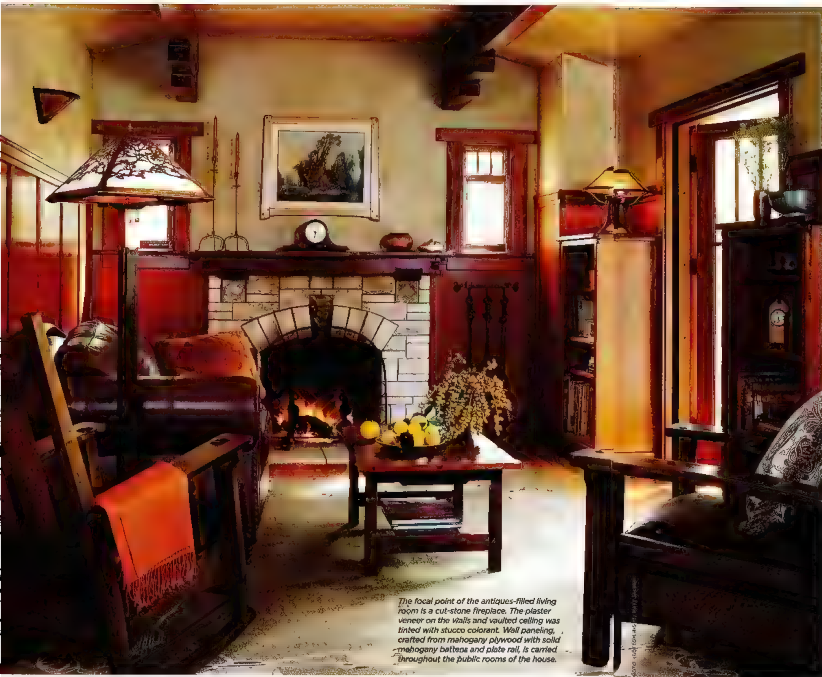
The elegant bracketed ceiling beams are in fact structural, made of engineered wood boxed in mahogany. They support the second floor.
