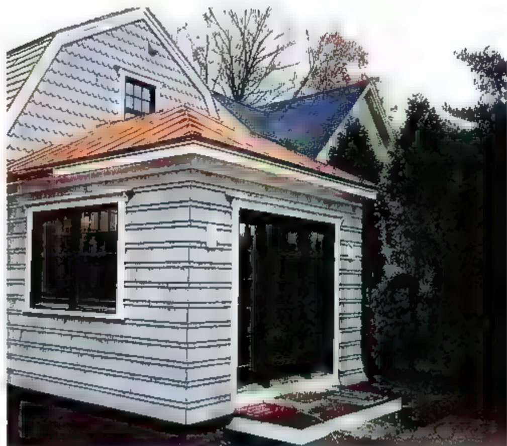
Ribbon coursing, the shingling technique used at the recent TV project house in Concord, Mass., creates distinctive horizontal stripes as it improves the walls' weathertightness.
