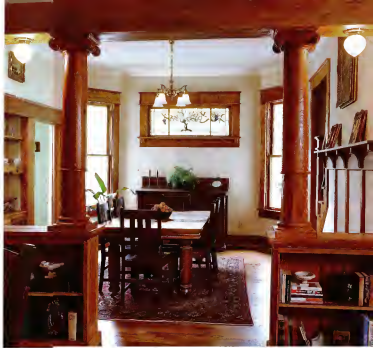
The dining room's beam-pile columns—refined of many coats of paint—are original to the house, as are the built-in bookcases, china cupboard, plate rack, and one-half of stained glass window that inspired the extensive renovation.
