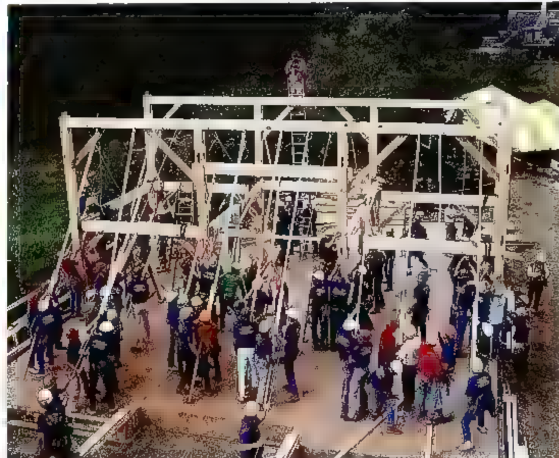
ABOVE: The original barn was deemed beyond saving for the homeowners' plans to convert it to a residence. RIGHT: Crew, students, and volunteers raise the timber frame of a new structure that will preserve the impression of a traditional barn. BELOW RIGHT: The timbers were first measured and drawn by computer and cut with power saws, then finished by hand by student timber framers.
