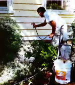
Steam Removal: developed in Canada to strip the finishes from gutters, it sprayed onto the clapboards by crew foreman William Gleason. Project contractor Jim Clark says, "If you're stripping your own house, keep an escape route open from a house until after you've sprayed all the siding and removed all the paint, just when the machine will under and you can see it again to paint the house."
