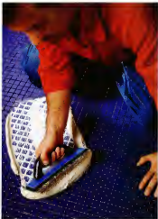
Grout is forced into the space between tiles with a rubber float called a float. The excess is wiped away with a wet sponge, leaving joints filled to just below the surface. After the grout goes rock-hard, the tiles are polished with a soft cloth to remove any "grout haze" left behind.
