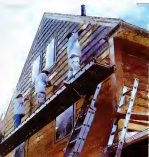
Blowdown: When left on overnight, the stripper leaves the paint on a surface off-white with a pebbly finish. After all the old paint is gone, the crew will give the house a quick sanding with 80-grit paper.
