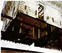
The house (top) and surrounding and boarded up for eight years. To make moving it more affordable, it was cut into five pieces and loaded onto trucks. The upper sections were lifted and lowered by cranes attached to steel I-beams (above and right).
