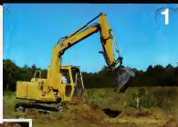
A FEW WEEKS LATER , the excavation contractor got to work. In a matter of minutes, he dug a narrow hole for the new septic tank, and in the first step in any septic system design, the soil at the proposed site must be evaluated. How it will absorb wastewater is first job. By observing the various layers and watching the dirt to a certain depth, he is able to determine things like, how wet it drains, and the location of the seasonal high-water mark, which establishes the limit of a leach field's depth.
