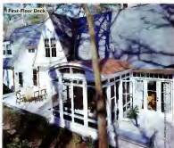
The basement-level deck (bottom left) is made with a plastic composite material, while the first-floor deck (above, and below right) is made with 100 percent plastic decking. Architect Jonnisch Ek's choice helps to keep the natural rainfall around in place.
